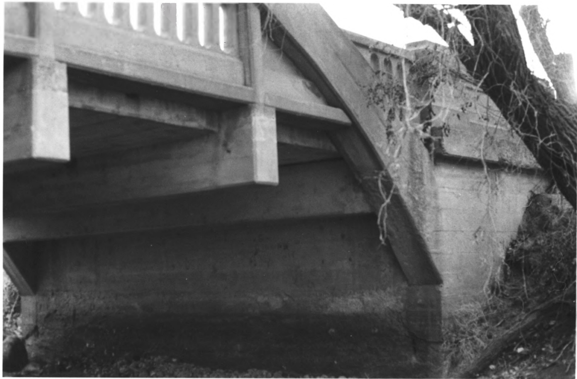
MILLER REE CREEK BRIDGE, HAND CO., SOUTH DAKOTA, No. 3
