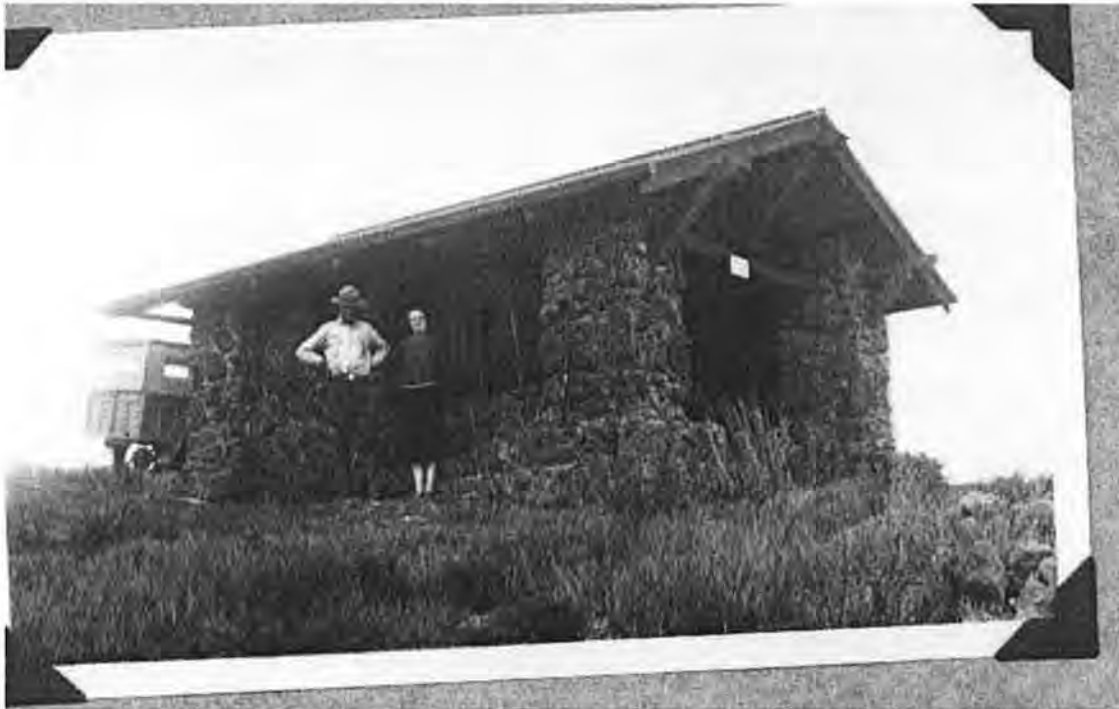
Fig. 1. Hilina Pali Picnic Shelter, 1931. Photographed by Merel Sager. Source: Landscape Architect Reports, Accession 370, Catalog #4959.
