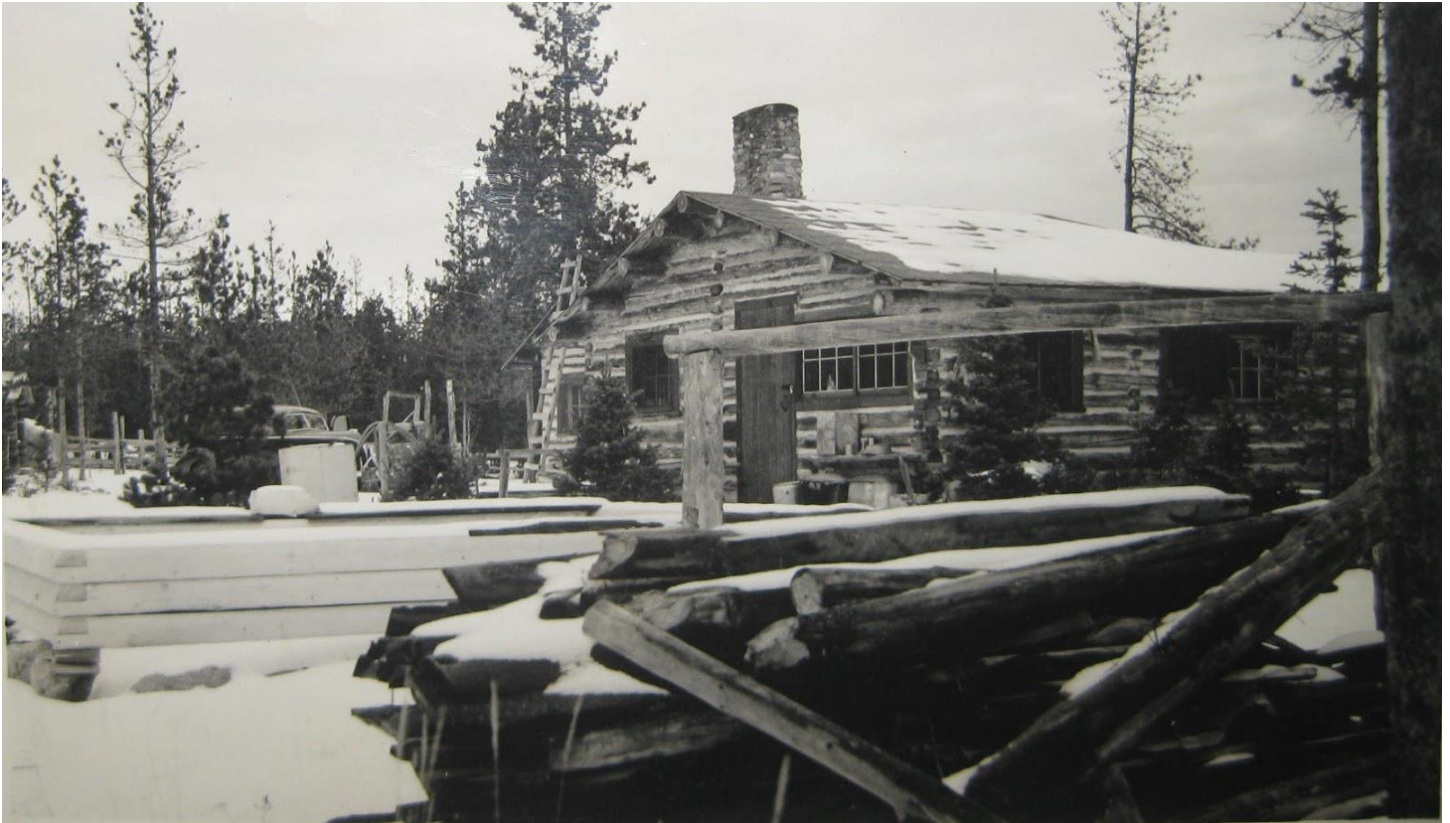
Photograph from 1939 showing construction of the Ice House.
