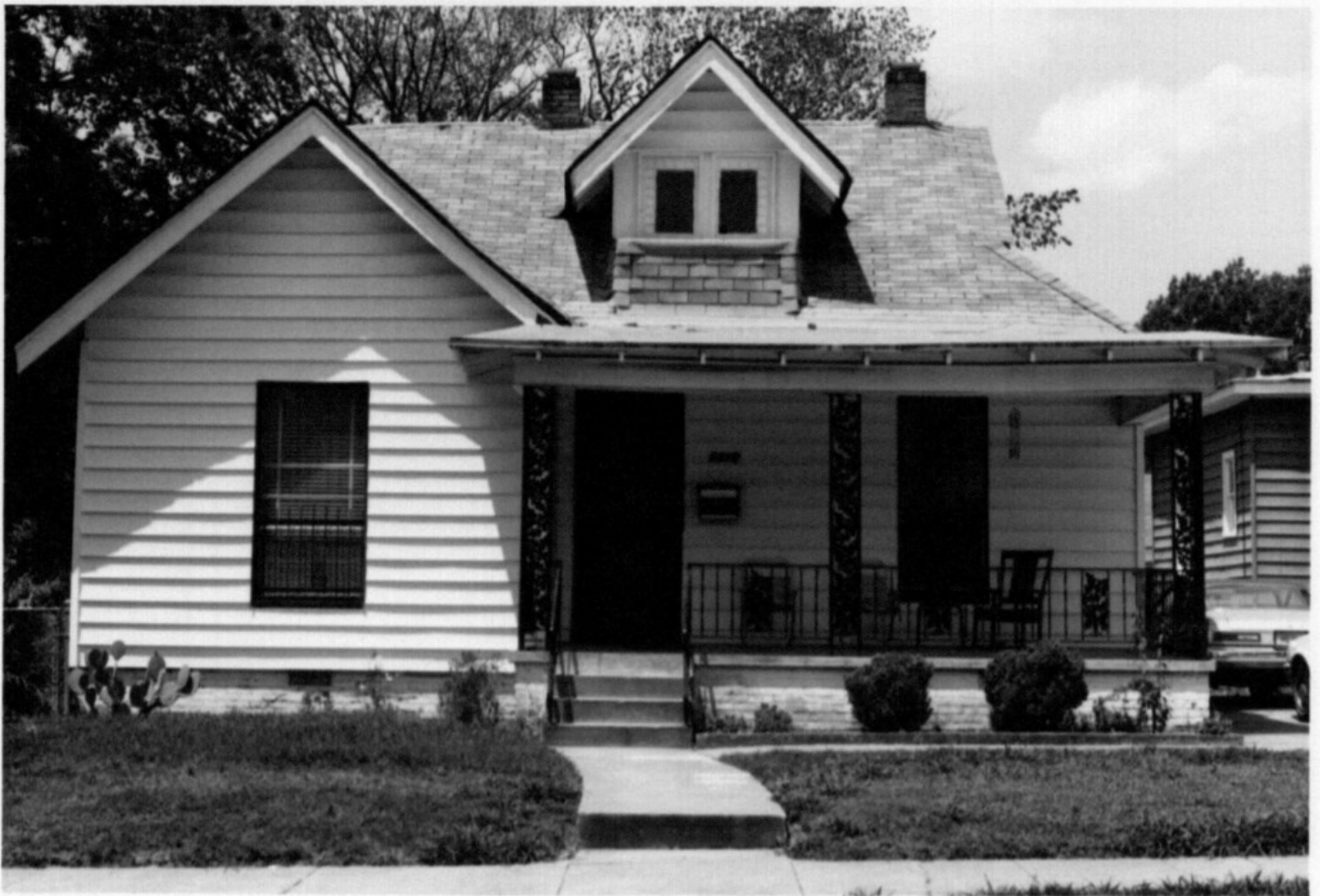
Figure 1: W. H. Vaughan Cottage – 1987.
