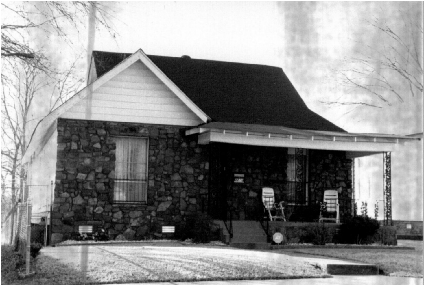
Figure 2: W. H. Vaughan Cottage – 1998.
