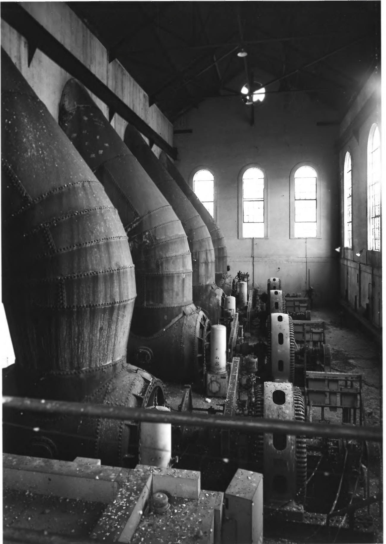
Plate 3 - S.U.M. Hydro - Electric Plant, interior, 1971 - Historic American Engineering Record.
