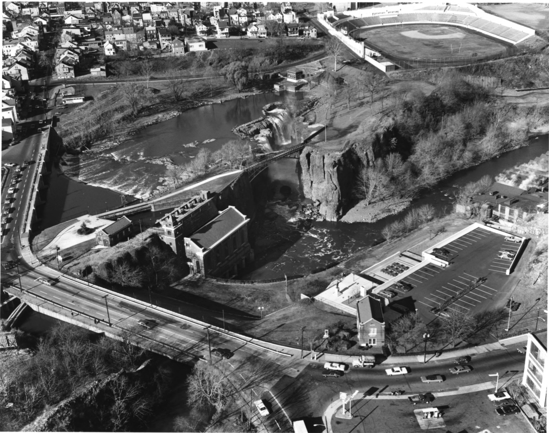
Plate 1 - General overview of Falls S.U.M. Dam and hydro-electric plant, Historic American Engineering Record.
