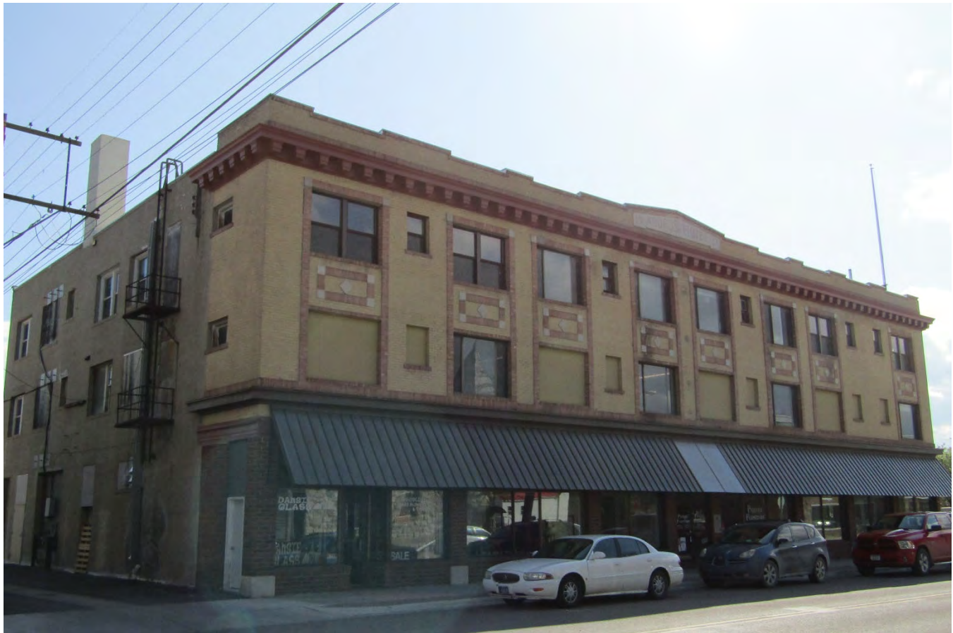
Description and view of camera: Andrus Hotel. Northwest (north) and Southwest (west) elevations, view to east.
