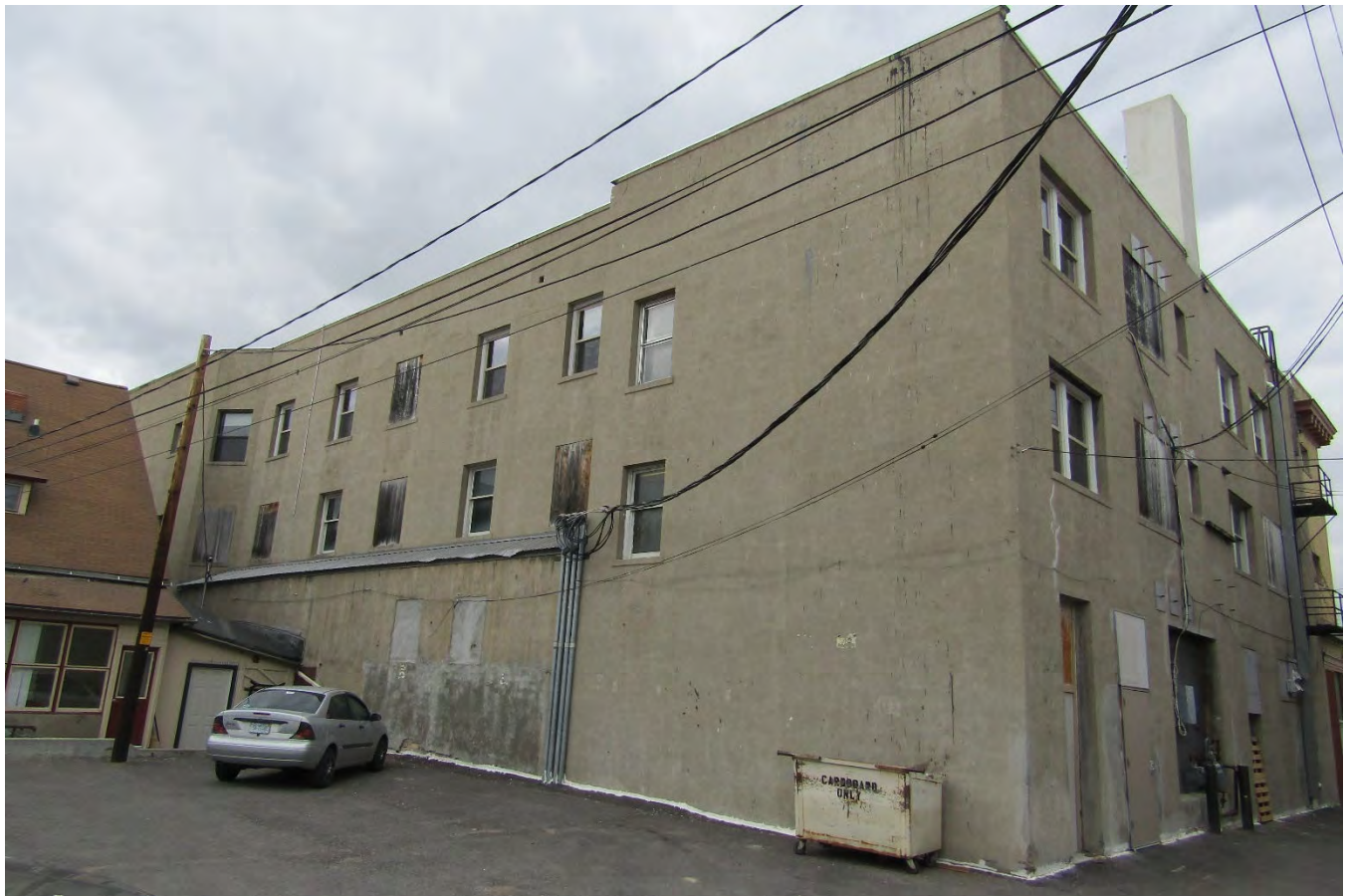
Description and view of camera: Andrus Hotel. Northeast (east) and Northwest (north) elevations. View to south. MT_BeaverheadCounty_AndrusHotel_0006
