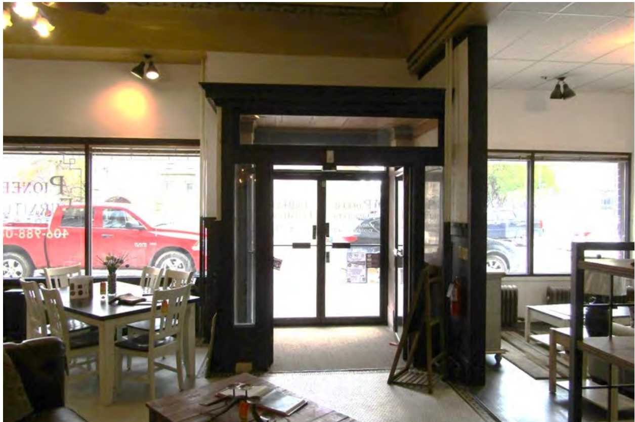
Description and view of camera: Andrus Hotel. Interior. Looking out toward original entry.
