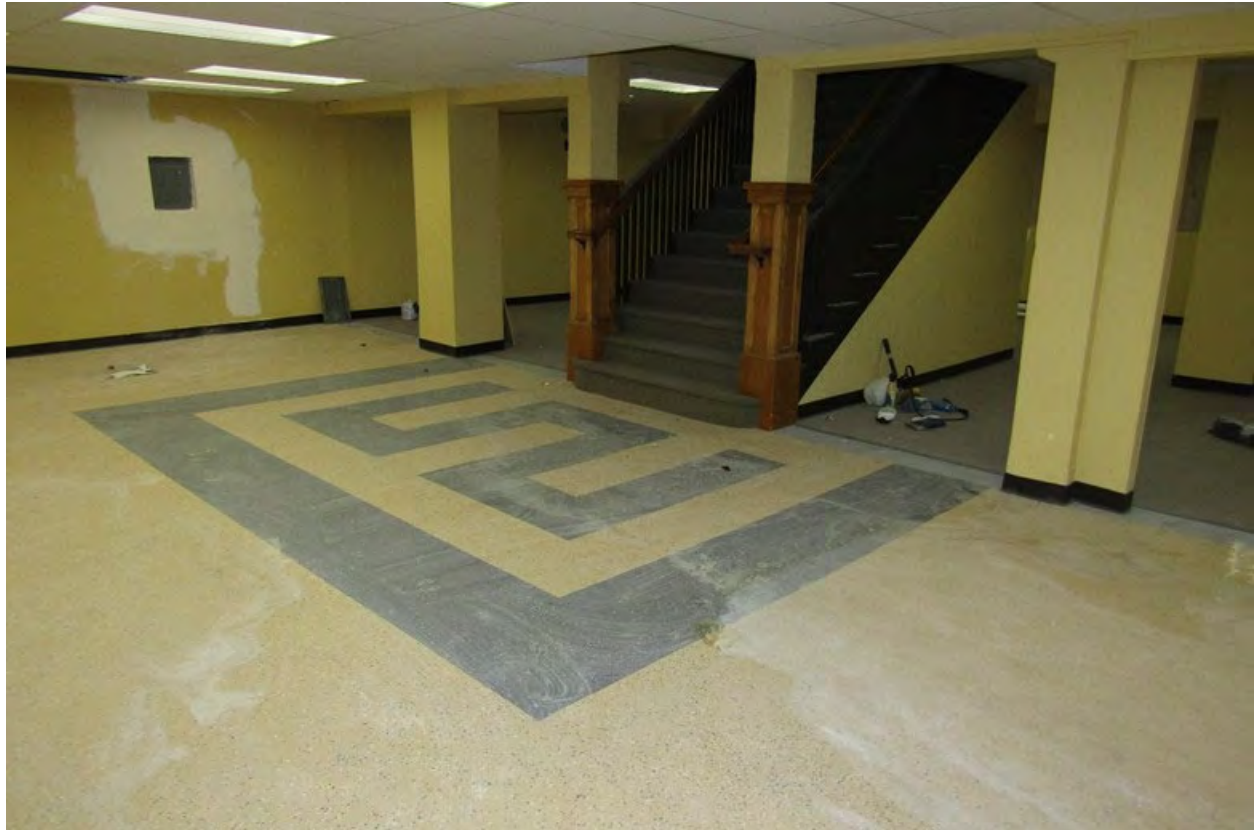
Description and view of camera: Andrus Hotel. Interior. Basement staircase and floor tiles.
