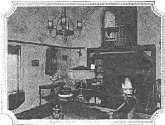
Fireplace and Balcony
