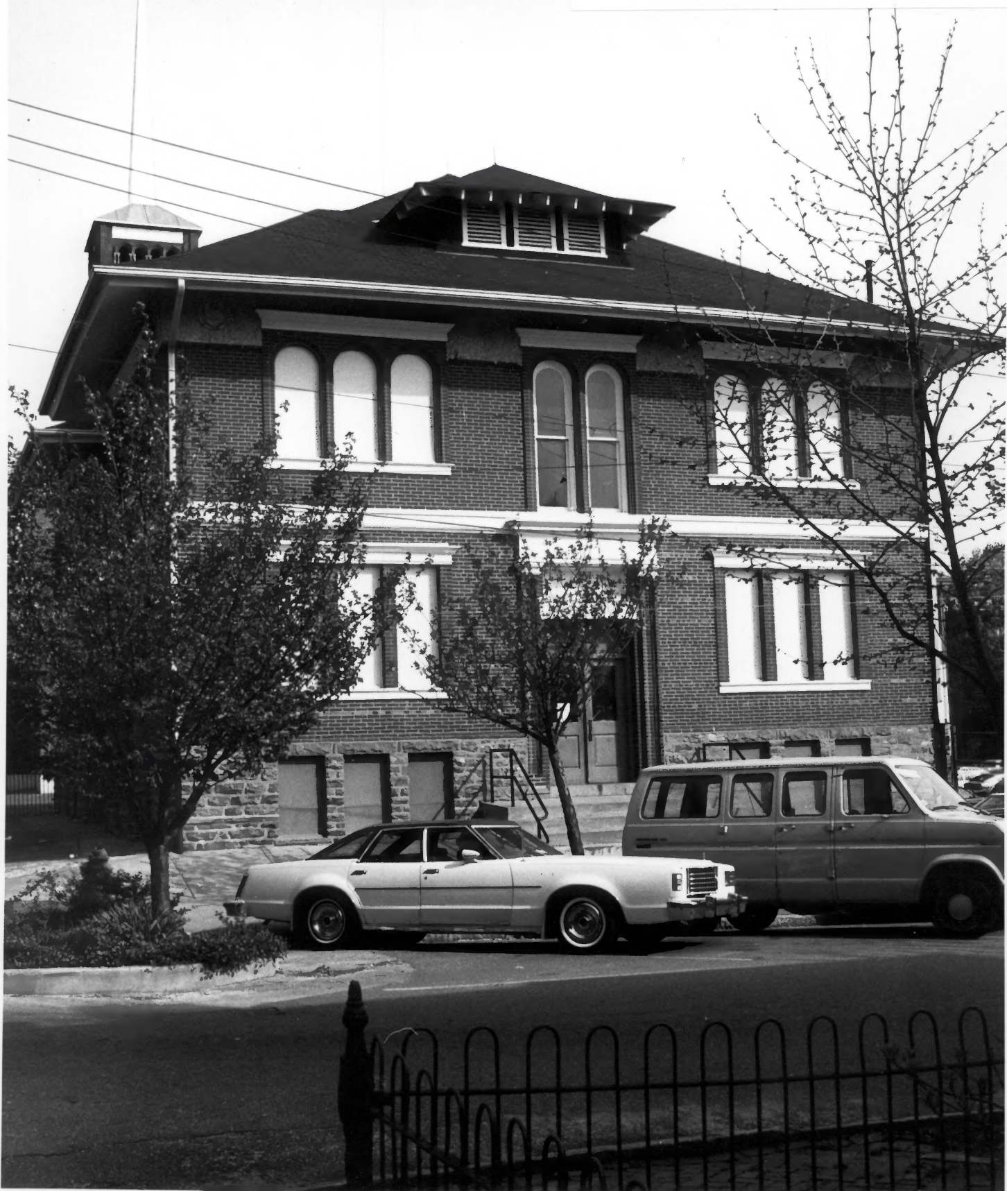
Shipley Run Historic District 900 Block North Monroe Street
