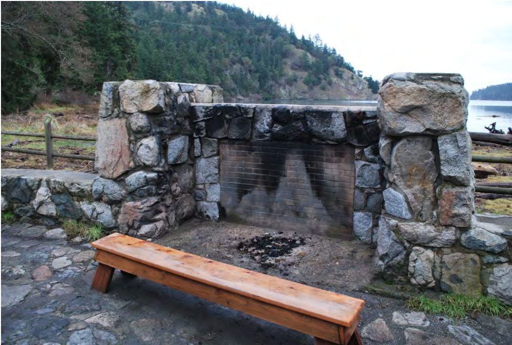
Photo 4 of 4: Cornet Bay Fire Circle, detail view of reflector taken 12/22/2014
