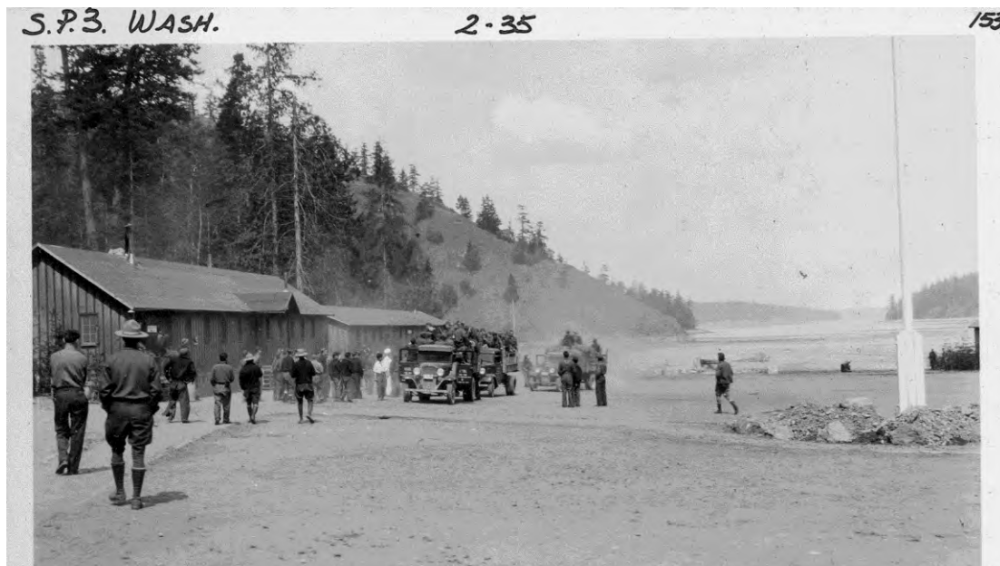
293 ARRIVAL ANOTHER GROUP OF ENROLLEES View of parade ground with Fire Circle under development in right background.
