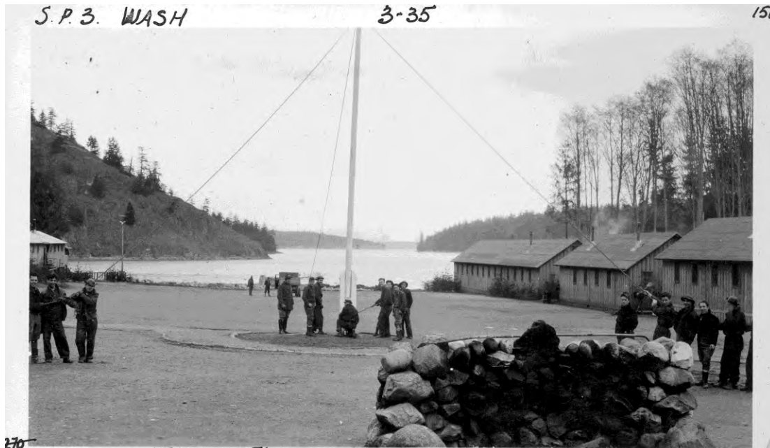
270 LOWERING CAMP FLAGPOLE TO INSTALL NEW ROPE View to northeast of CCC Camp SP-3 parade ground, Fire Circle visible behind flag pole.
