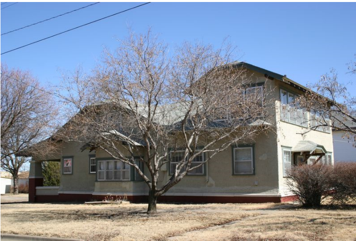
(Above) 238 W Wisconsin (side and rear elevations), Russell, Russell County, KS.
