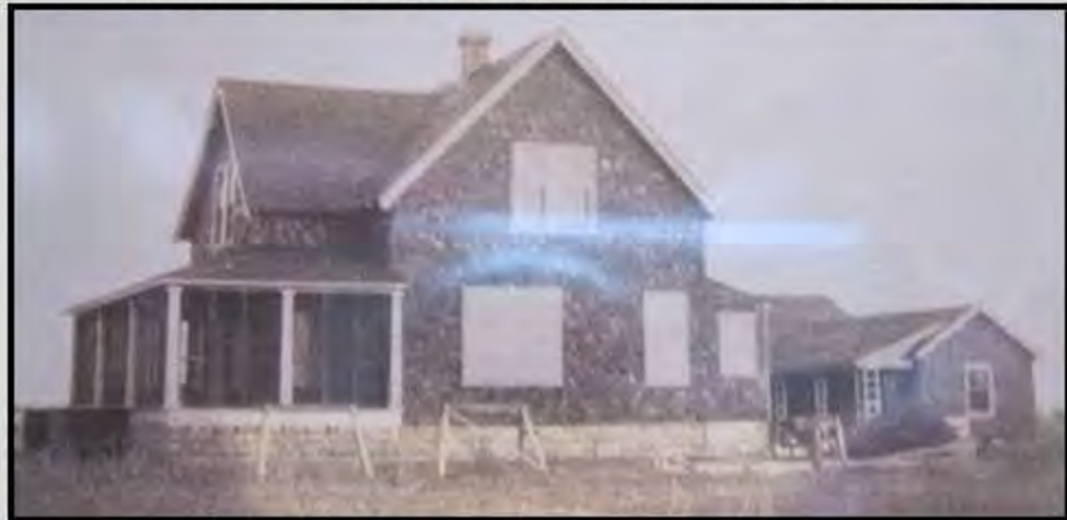
c. 1927 – 1930 view of cottage re-sheathed with cut shingles
