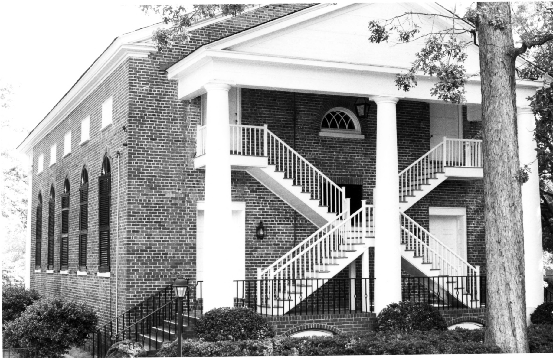
Bethesda Presbyterian Church Kershaw County, South Carolina 5/31/84 North (Rear) Facade
