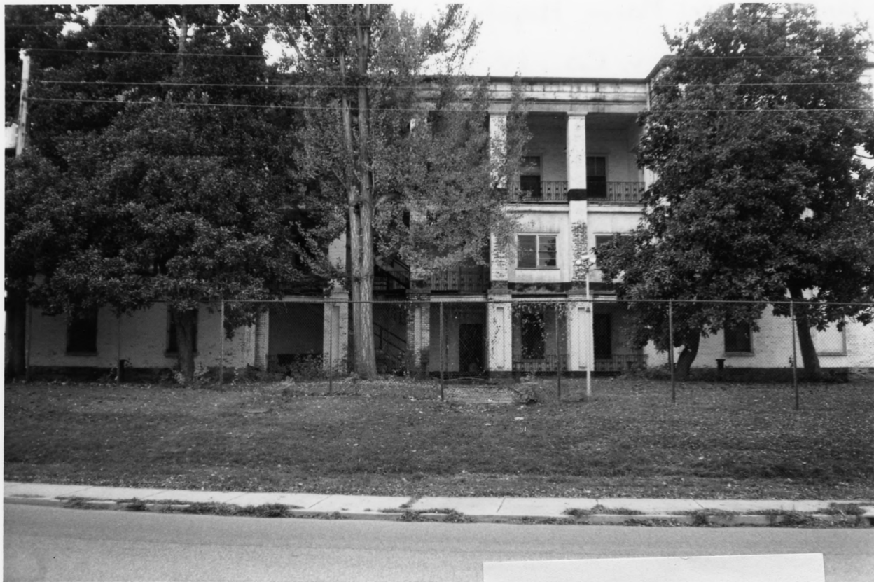
U.S. MARINE HOSPITAL Louisville, Kentucky North facade Photo: Carolyn Brooks, 1995
