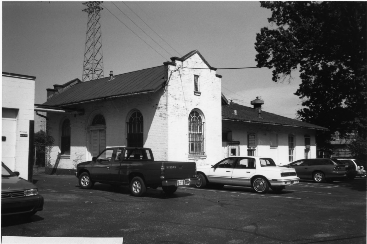
U.S. MARINE HOSPITAL Louisville, Kentucky Laundry Photo: Carolyn Brooks, 1996
