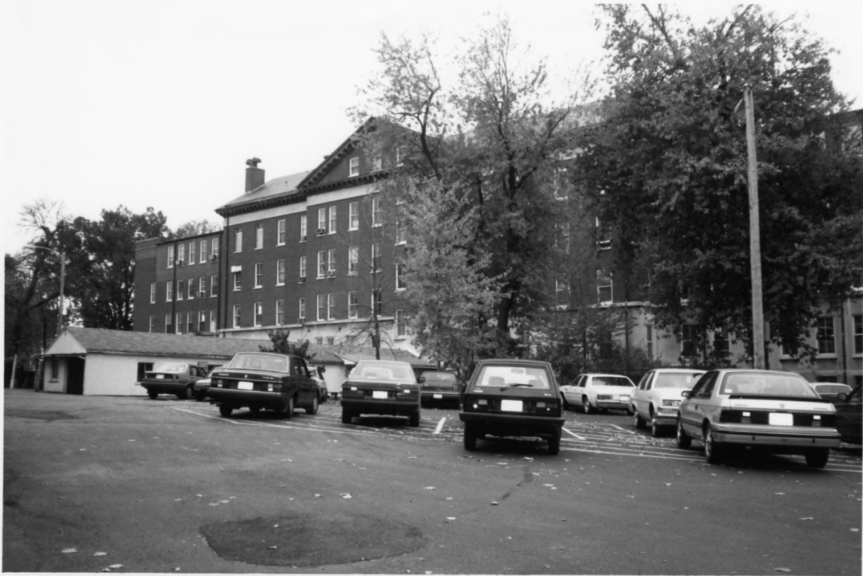
U.S. MARINE HOSPITAL Louisville, Kentucky North facade of 1933 hospital Photo: Carolyn Brooks, 1995
