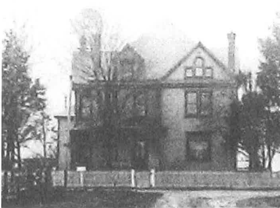
Fig. 8 – Original North façade (1930) camera facing south
