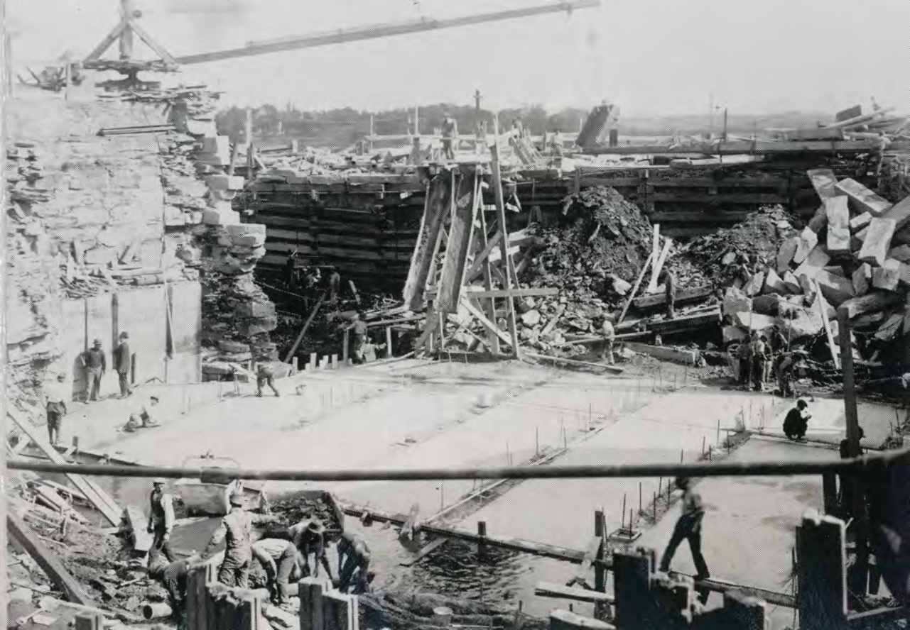
Photograph 2 Rebuilding of headgate substructure 1914
