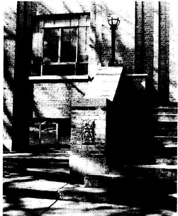
Courthouse with original windows in 1983
