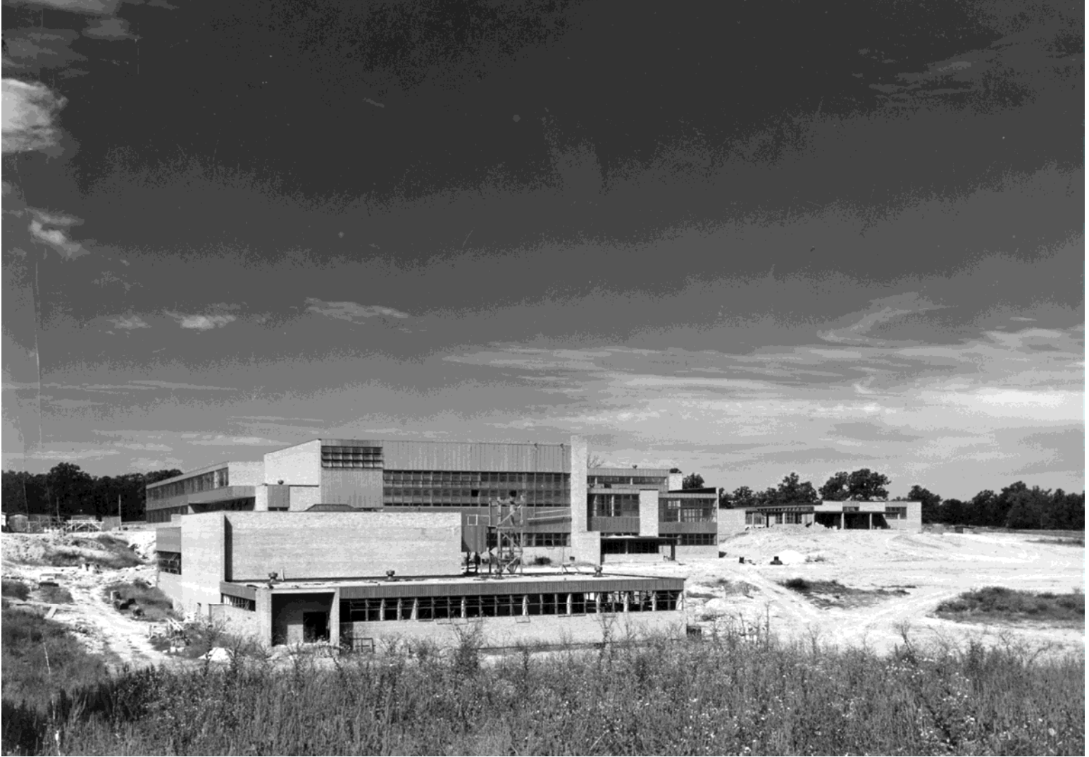
Figure 4: BTW HS Under-construction September 1949 (Photographer: H.O. Wiseman)
