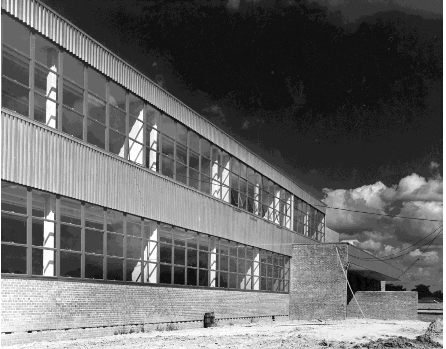
Figure 5: BTW HS Finishing Construction September 1949 (Photographer: H.O. Wiseman)
