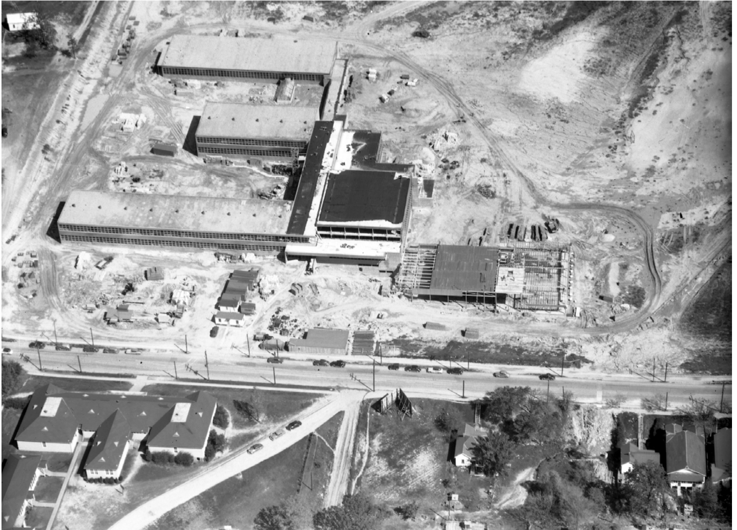
Figure 1: BTW HS Under-construction Aerial View ca1949-1950.
