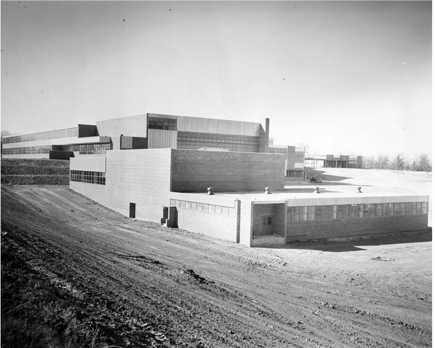
Figure 6: BTW HS Finishing Construction ca1949-1950 (A)
