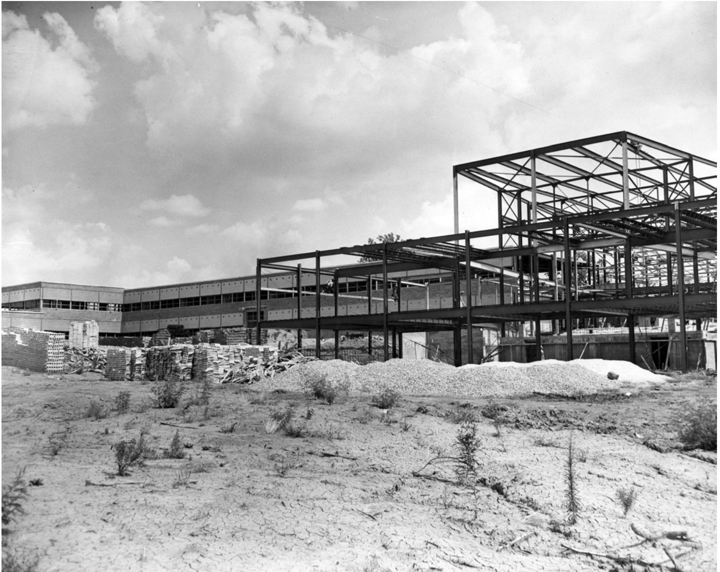
Figure 2: BTW HS Under-construction ca1949-1950 (A).
