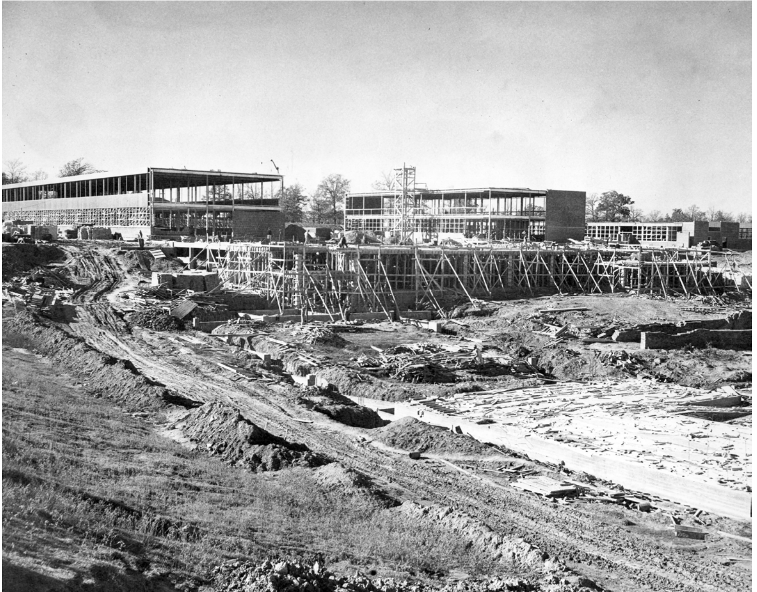
Figure 3: BTW HS Under-construction ca1949-1950 (B)
