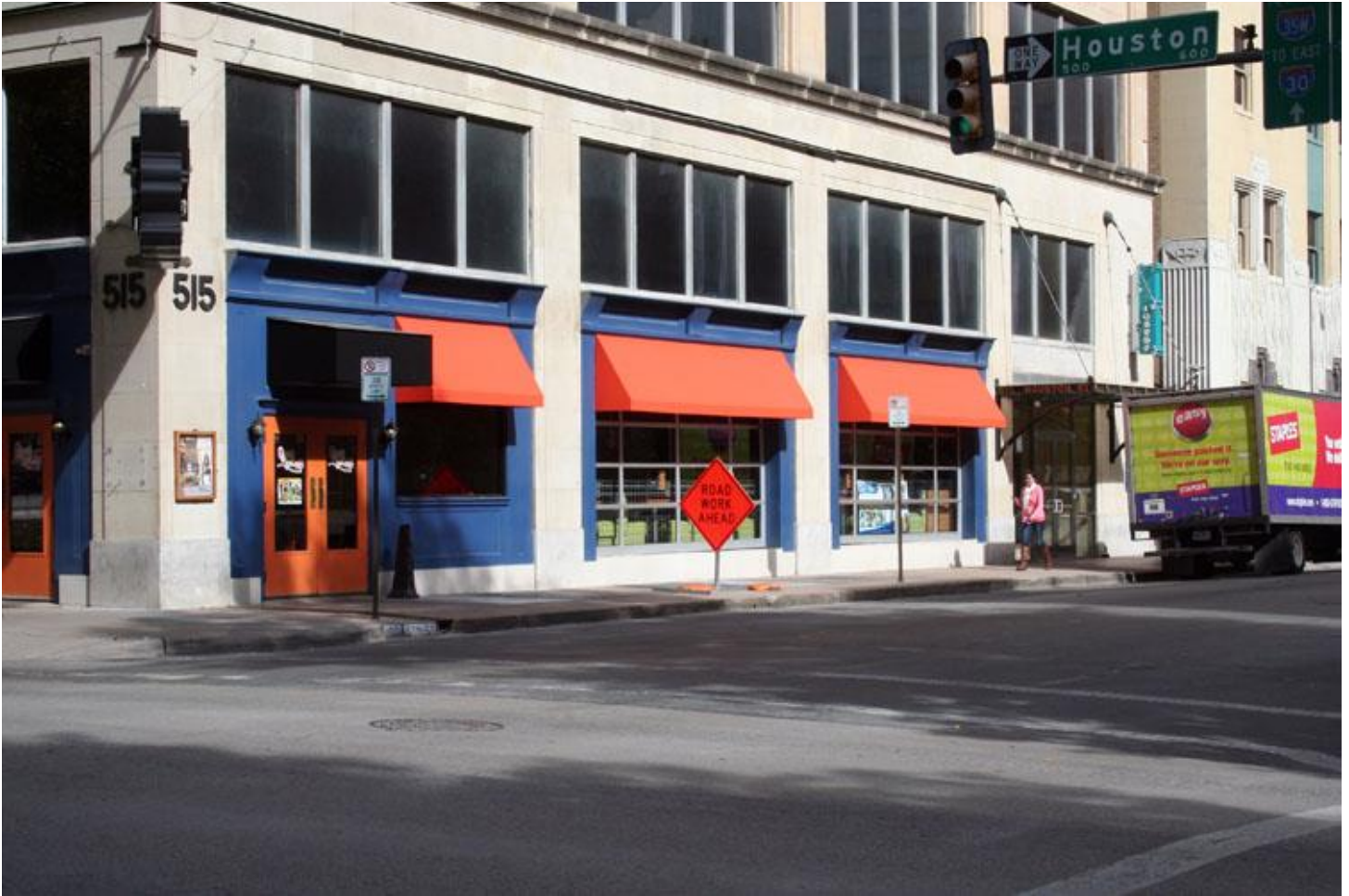
Photo 3: View of south elevation, detail of ground floor storefronts, looking east
