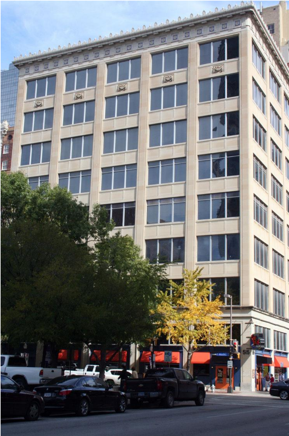
Photo 6: View of west elevation, looking northeast
