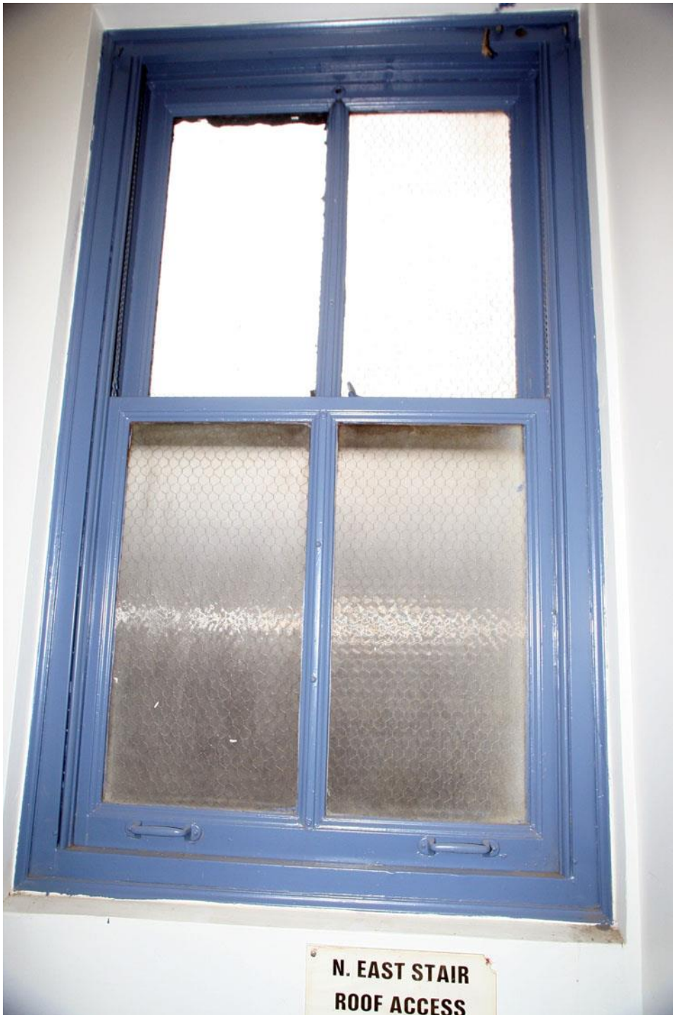
Photo 16: Second floor, detail of window, looking east
