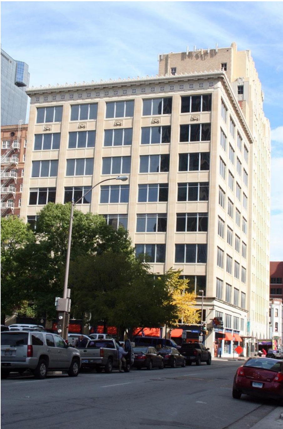
Photo 1: View of west and south elevations, looking northeast
