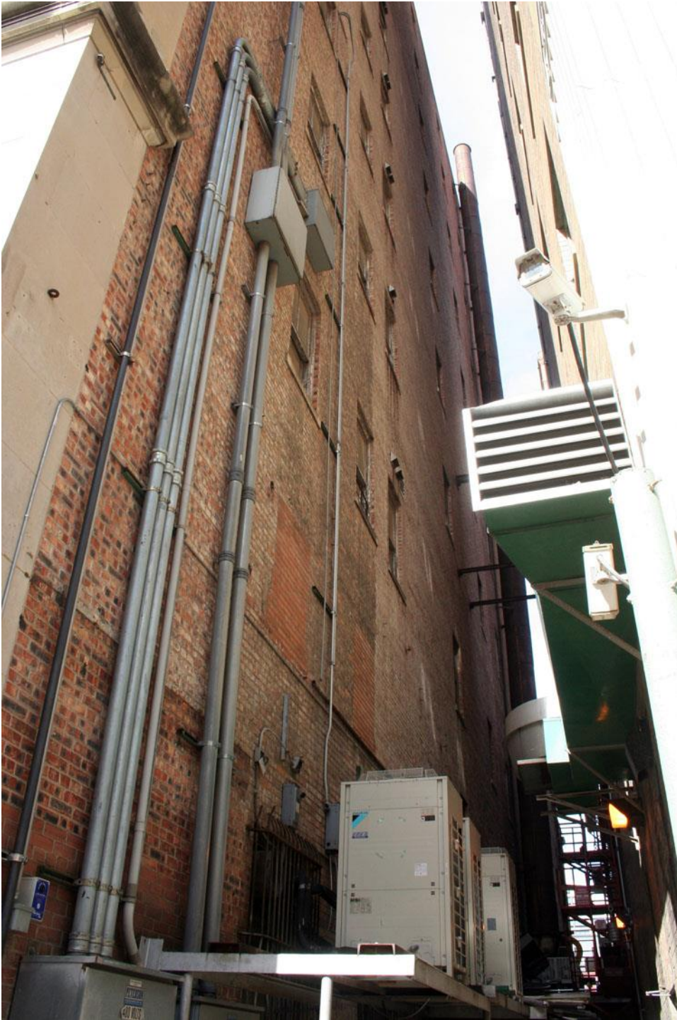
Photo 5: View of east elevation, looking north
