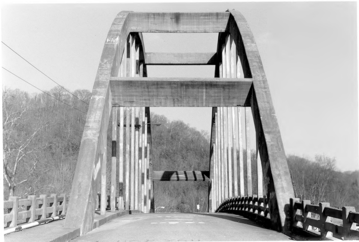
West Prestonsburg Bridge Prestonsburg MS Floyd Co, KY
