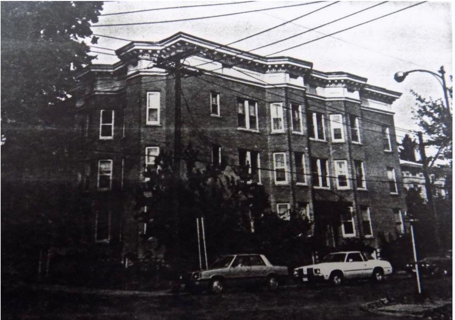
Figure 5. Abingdon Apartments, ca. 1980s Source: Nostalgic Watertown NY
