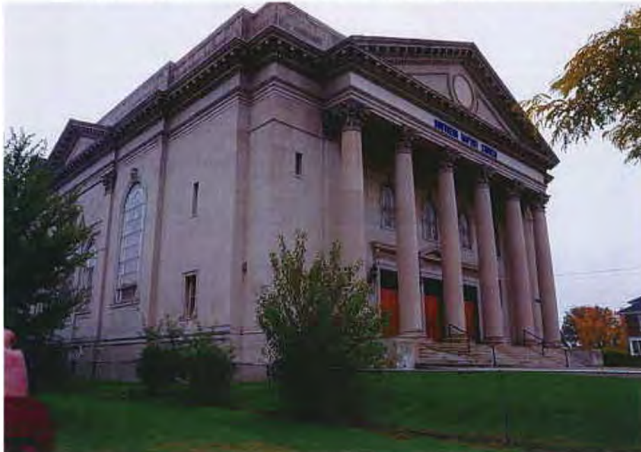
Figure 16. Former Adath Israel Temple (1926) 3556 Reading Road, Cincinnati (Beth Sullebarger, June 6, 2018)
