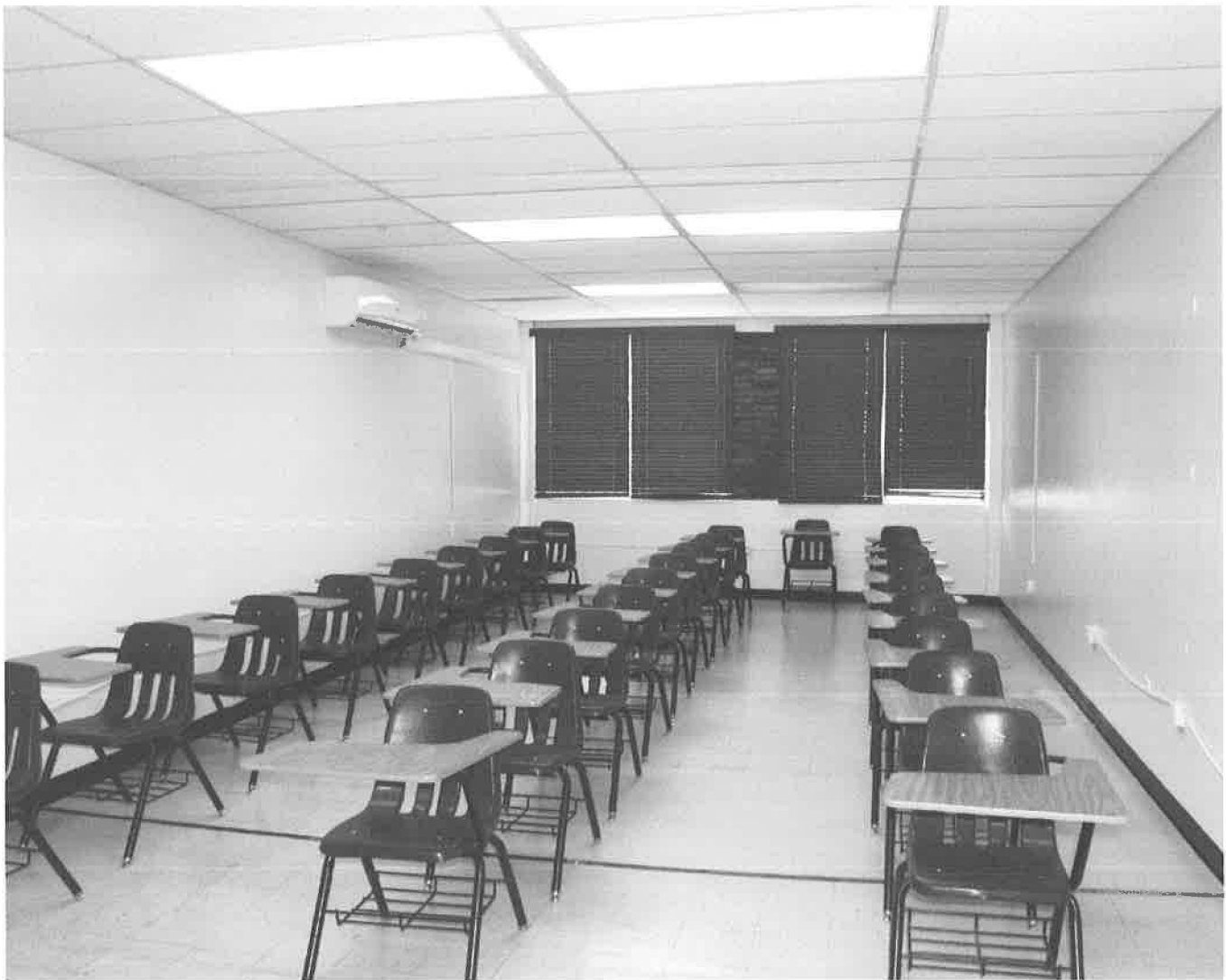
Fig.7. In 1951, many of the empty bays at the second floor were proposed as offices. These rooms are now used as classrooms. They have kept the original spatial layout, the set of glass windows and the clay brick pier. These spaces, as indicated in Little's plans, were to have acoustical tiles in the ceiling, vinyl tiles flooring, and cement plastered walls, which they still have.
