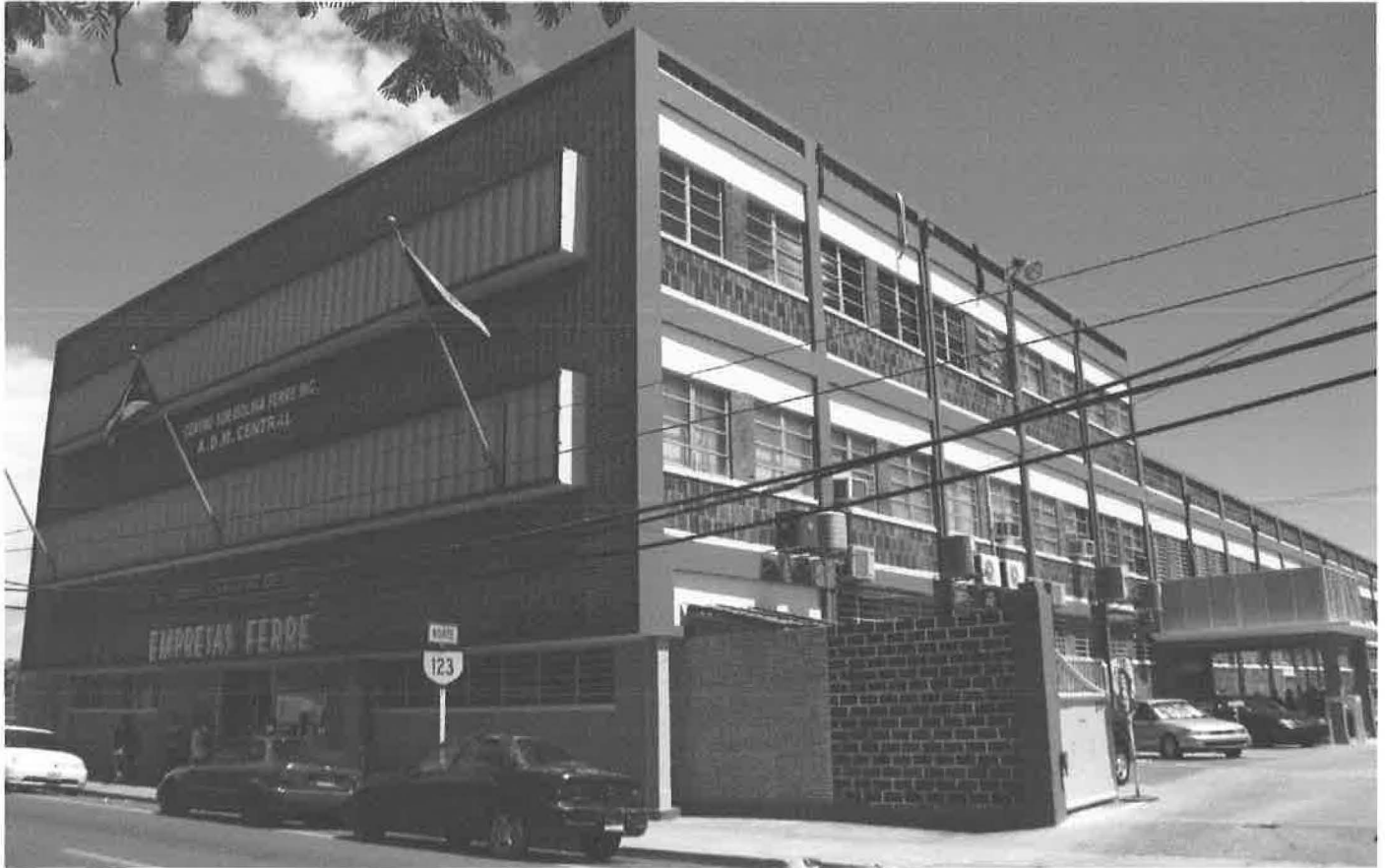
Fig.1. Edificio Empresas Ferré's main façade and partial view of South elevation.
