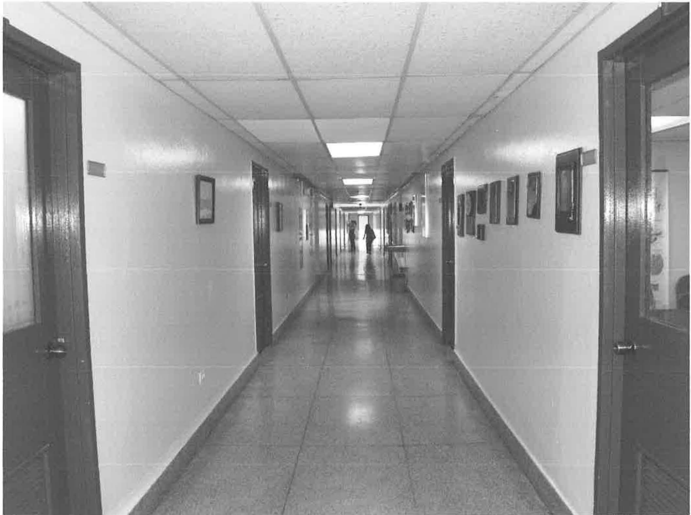
Fig. 8. In 1951, this section of the second floor was planned and layout as future offices. Today they are use as classrooms. The corridor has the original terrazzo floor, and the ceiling still made of acoustical panels, as planned. Two original skylights allow for direct sunlight into the corridor.
