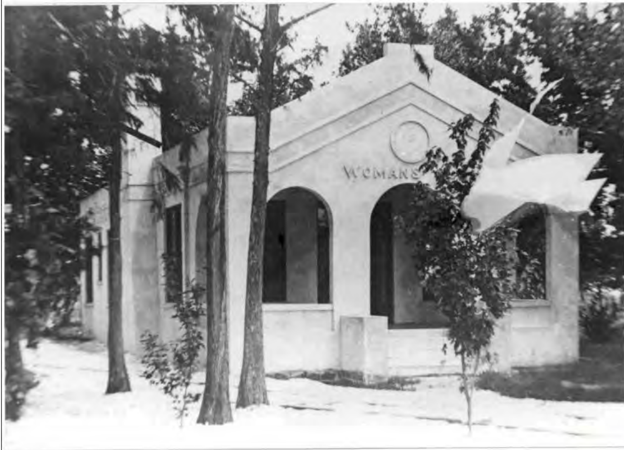
Figure# 4: Scan of photo of the original 1917 main (west) entrance, showing original arcaded porch. Fort Lauderdale Historical Society.
