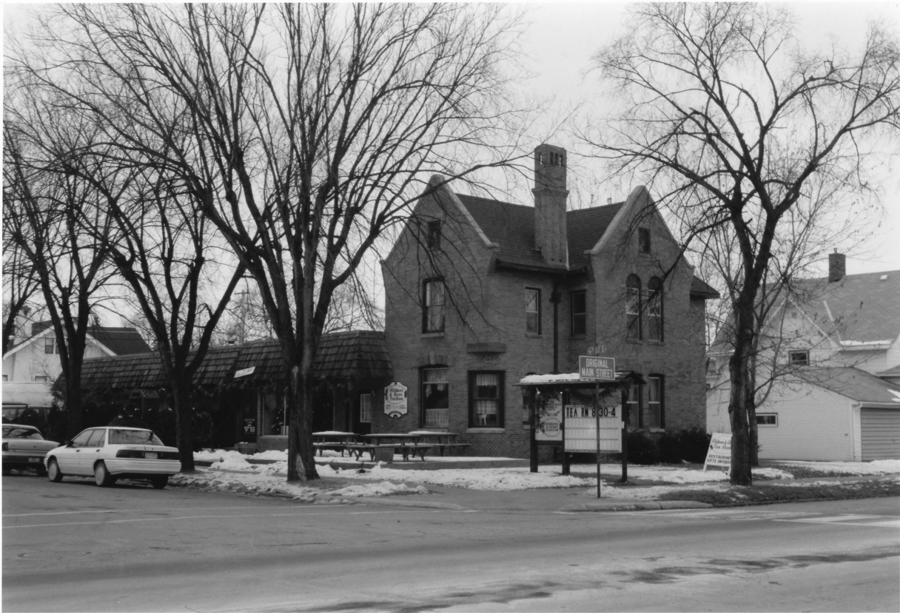
House #12 Original Main Street Historic District Stearns Co. MN 011496 | 15
