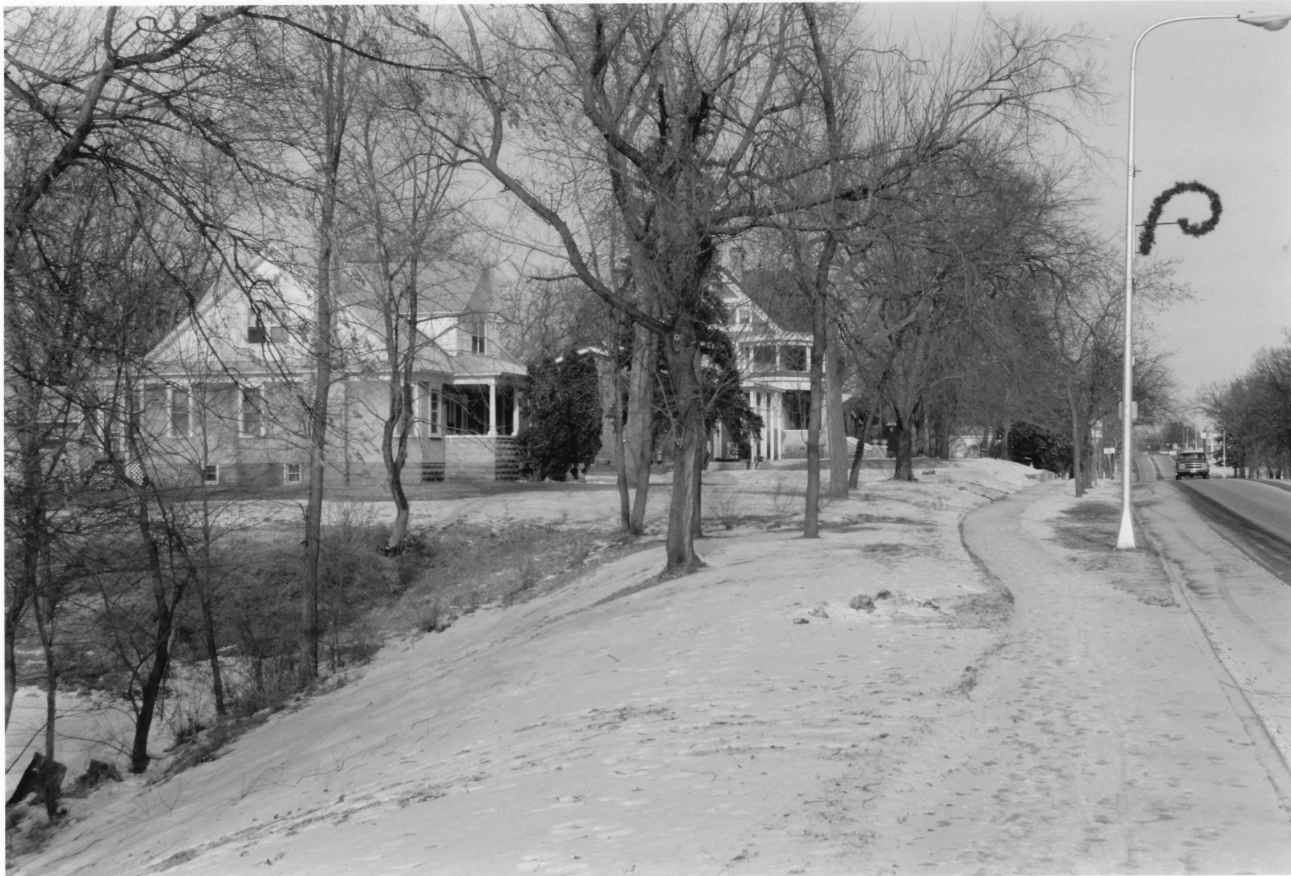
Streetscape- Looking at the west side of North Main Street between Sawk River and North First Street Original Main Street Historic District Stearns Co., MN 011483- 6A/6
