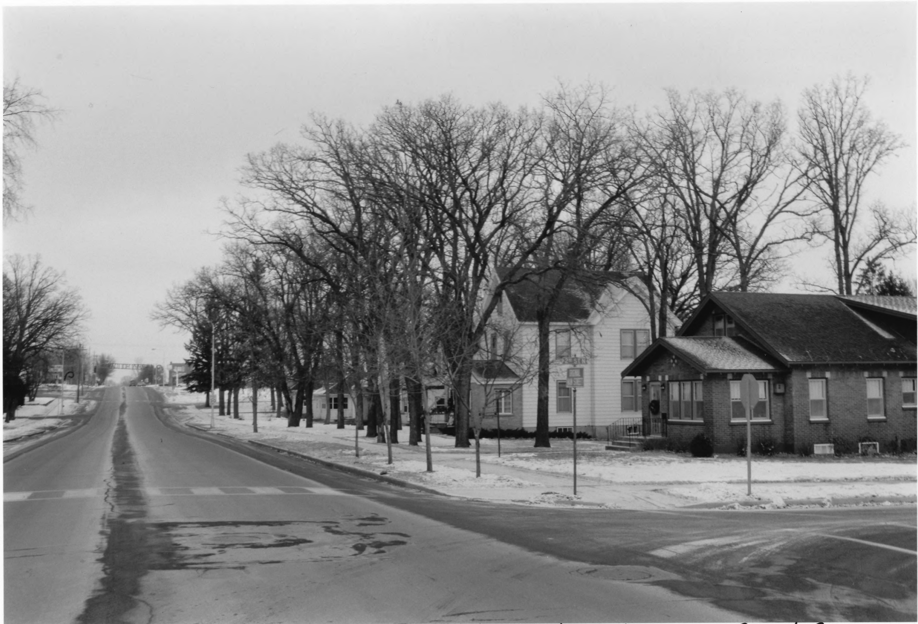
Streetscape- Looking at the east side of the 600 Block of North Main Street from South Seventh Street Original Main Street Historic District Stearns Co., MN 011483 - 24A
