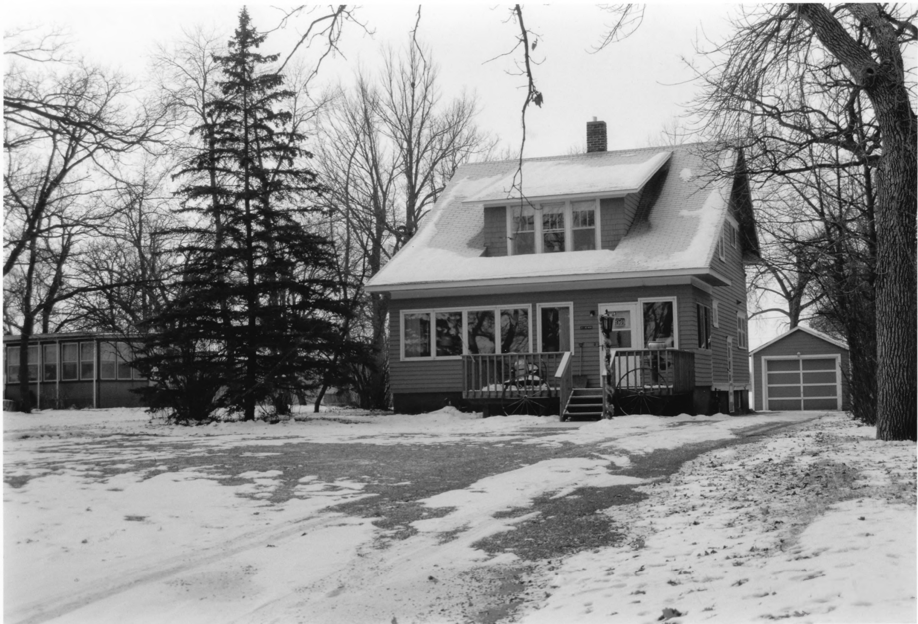
House, #99 Original Main Street Historic District Stearns Co., MN 011480 - Z1A
