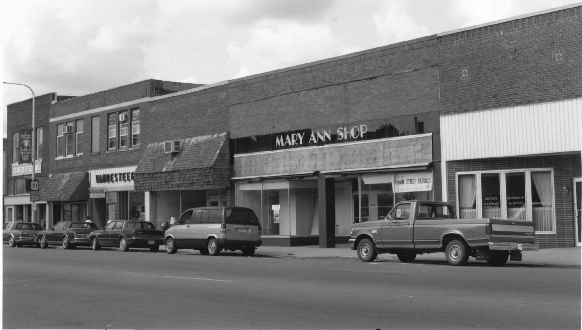
Streetscape: Looking southwest at west side of Main Street from Sinclair Lewis Avenue Original Main Street Historic District Stearns Co., MN 87843 - 12A/13 (Hess-Roise)
