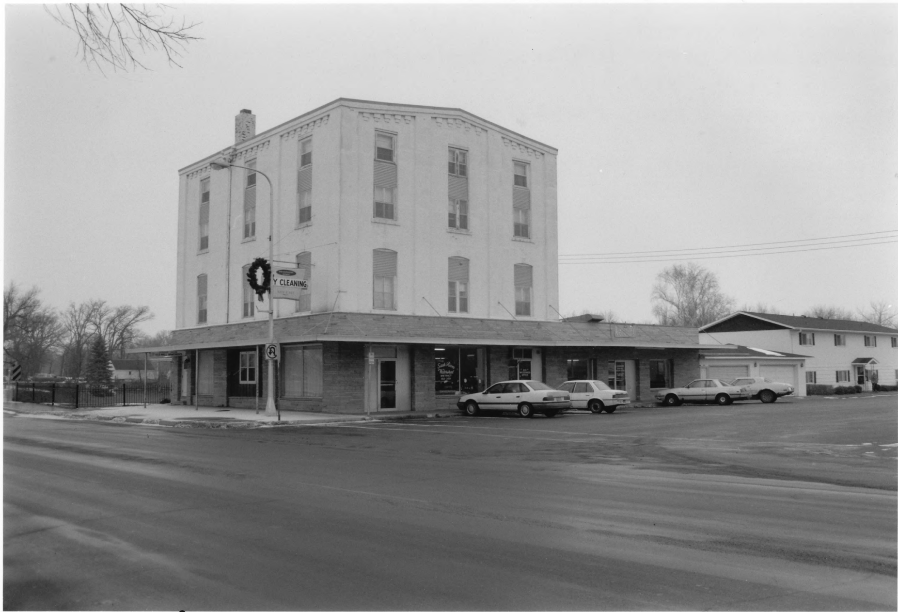
Central Minnesota Power and Milling Company Flour Mill, # 75 Original Main Street Historic District Stearns Co., MN 011491-21
