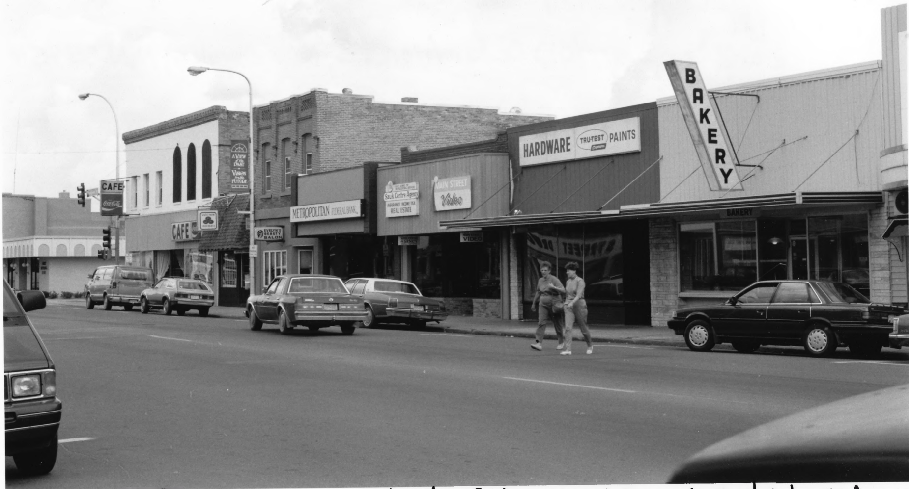
Streetscape: Looking northeast at east side of Main Street toward Sinclair Lewis Avenue Original Main Street Historic District Stearns Co., MN 87843 - 22A/23 (Hess-Roise)
