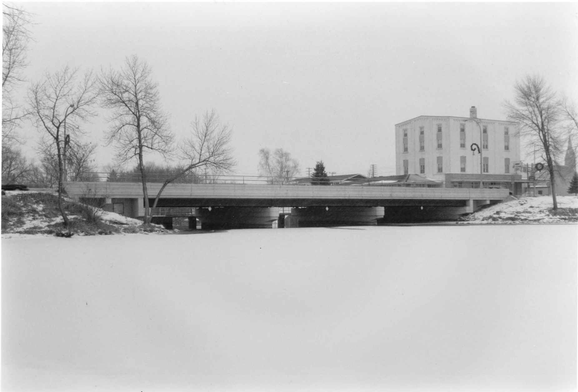
Center-Bridge No 5428 (non-contributing), Right-Central Minnesota Power and Milling Company Flour Mill Original Main Street Historic District Stearns Co., MN 01485 - 3A/4
