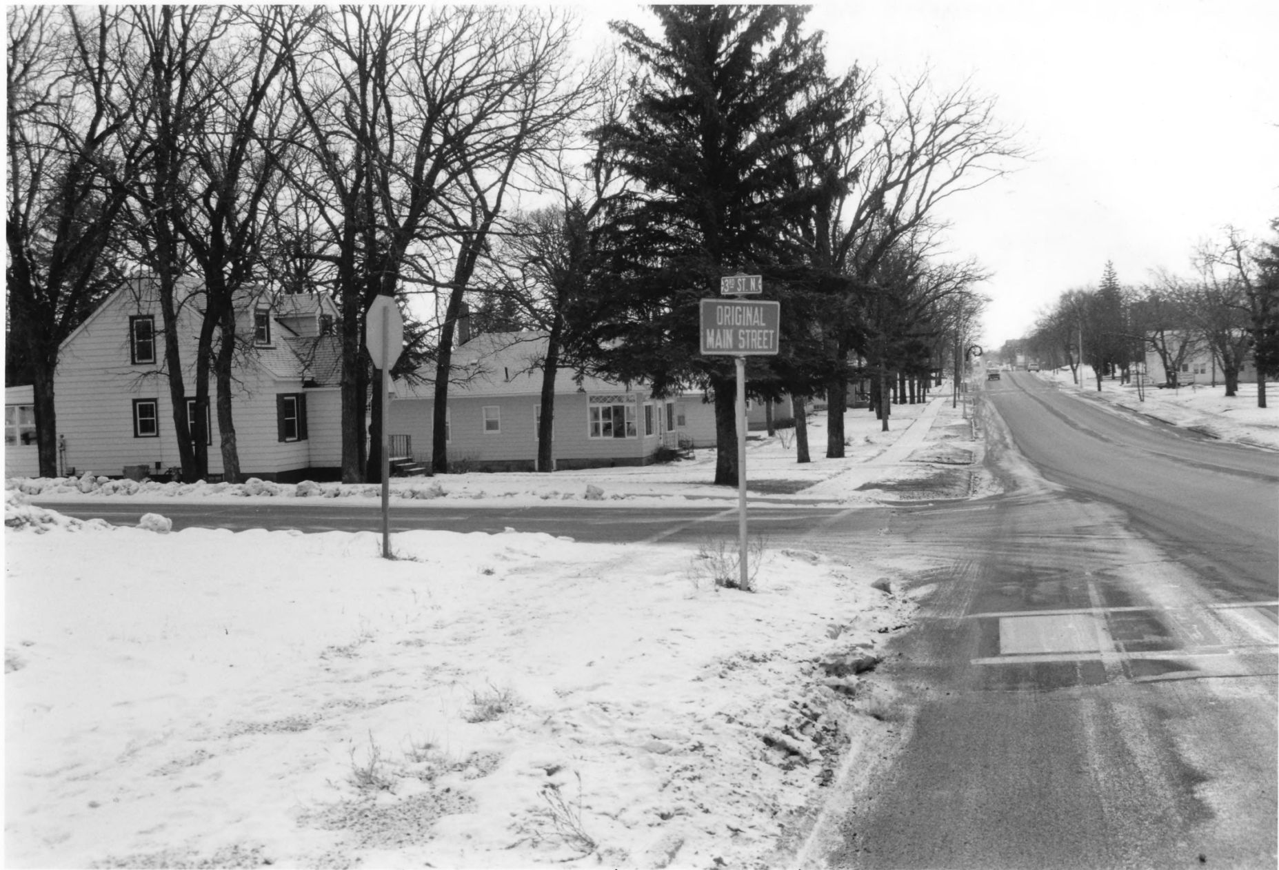
Streetscape - Looking at the east side the zoo Block of North Main Street from North Third Street Original Main Street Historic District Stearns Co., MN 011480 - 9A
