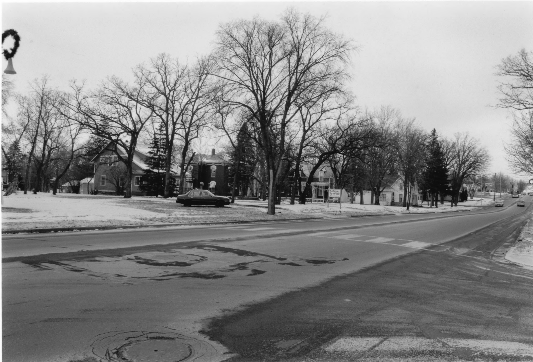
Streetscape: Looking at the west side of the 200 Block of North Main Street Original Main Street Historic District Stearns Co., MN
