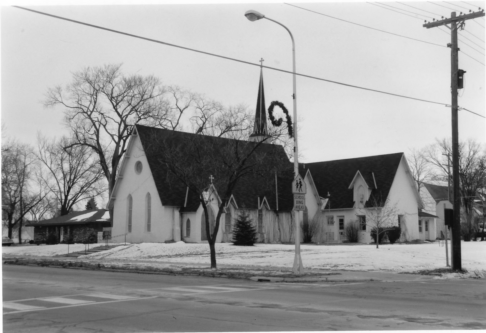
Church of The Good Samaritan #20 Original main Street Historic District Stearns Co. mn 011486 / 5A / 6
