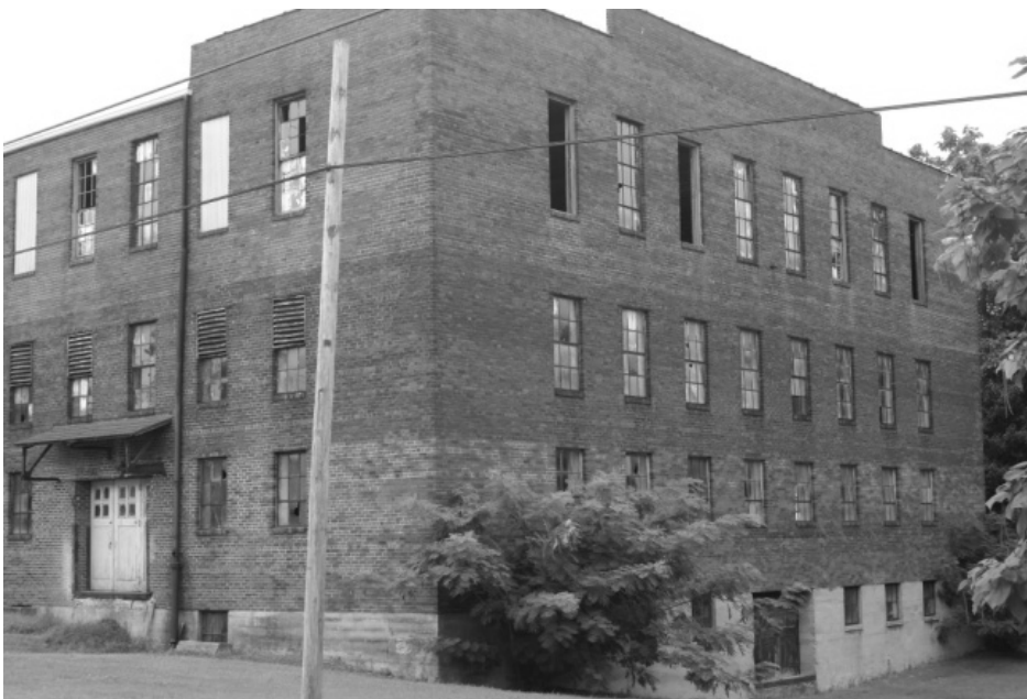
Rear of the W.G. Swann building ( Angela Rowlett Lampe )
