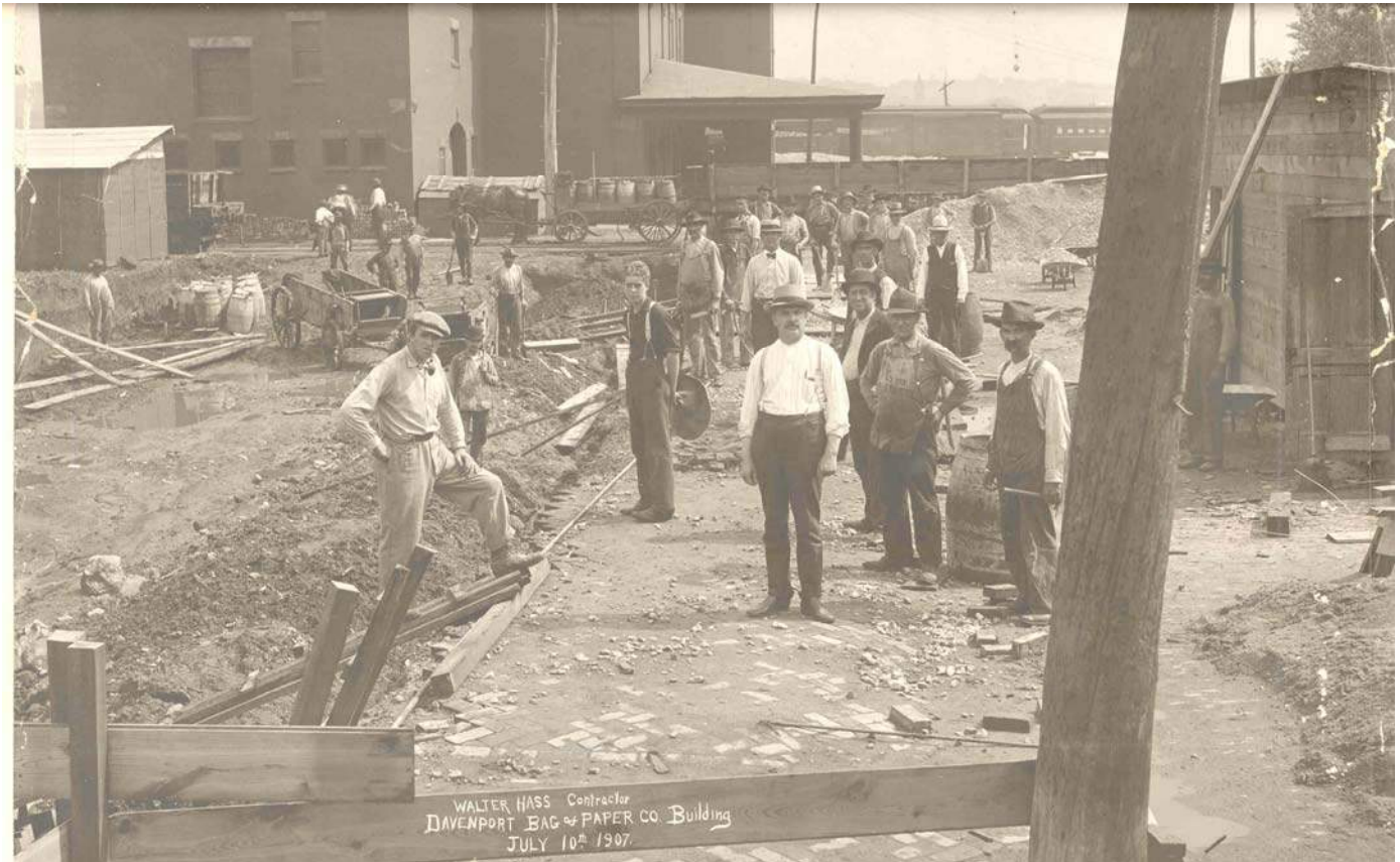
Construction beginning, July 10, 1907
