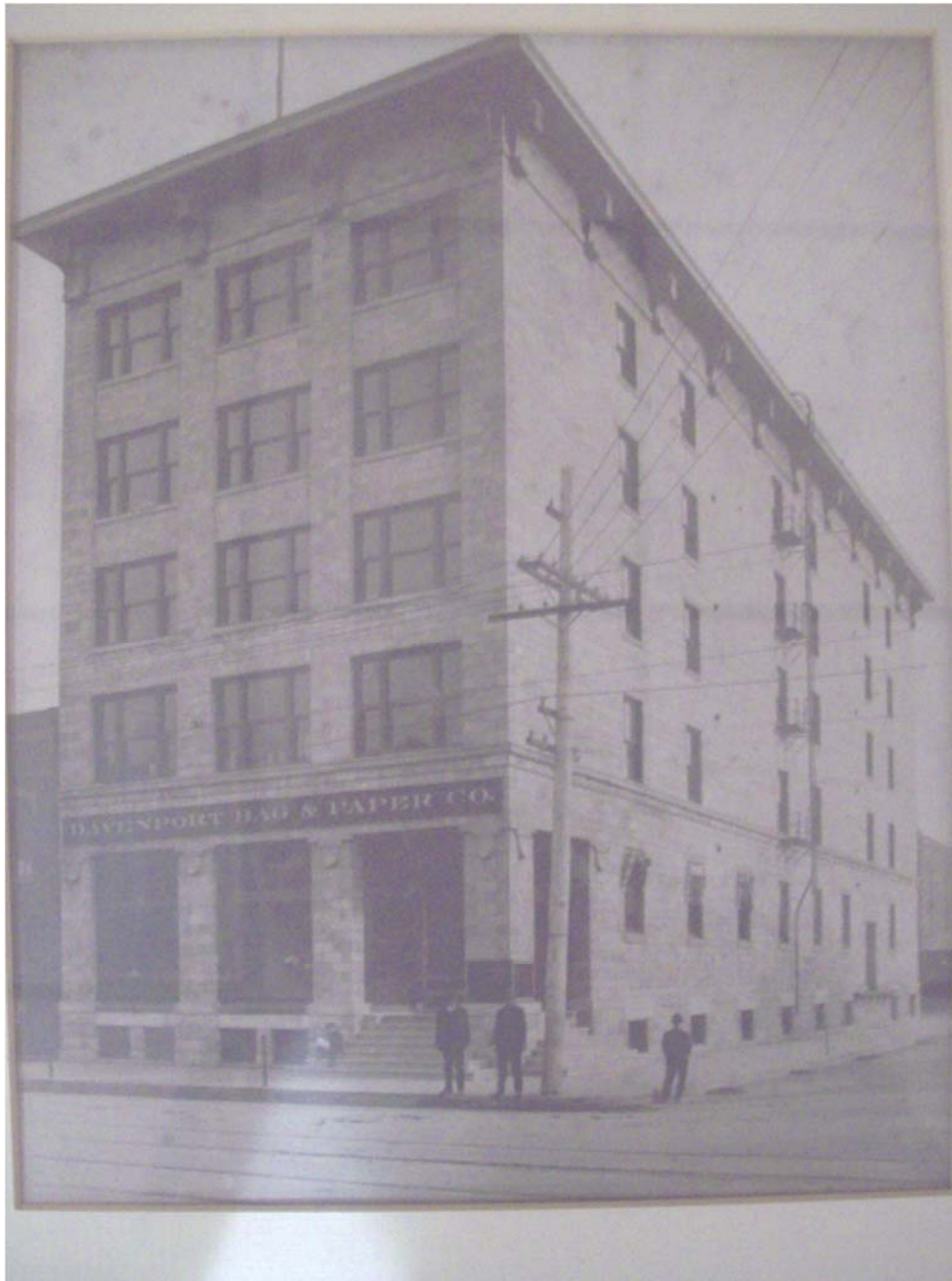
Construction complete, ca. 1908, looking south. See original cornice, which was rebuilt ca. 2014, constructed entirely of metal. (Source: Valley Construction Company, April 2014)
