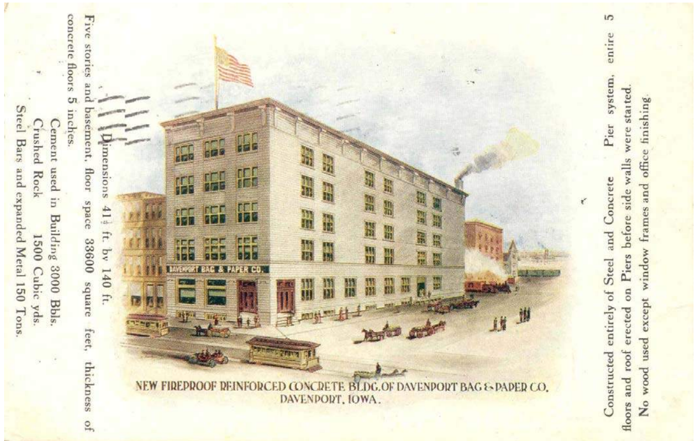
This postcard image from 1907 documents the “New Fireproof Reinforced Concrete Bldg. of Davenport Bag & Paper Co.” Notice that the building of today looks much as it did when constructed. This image also serves to document the building’s original streetscape. (View to South)
