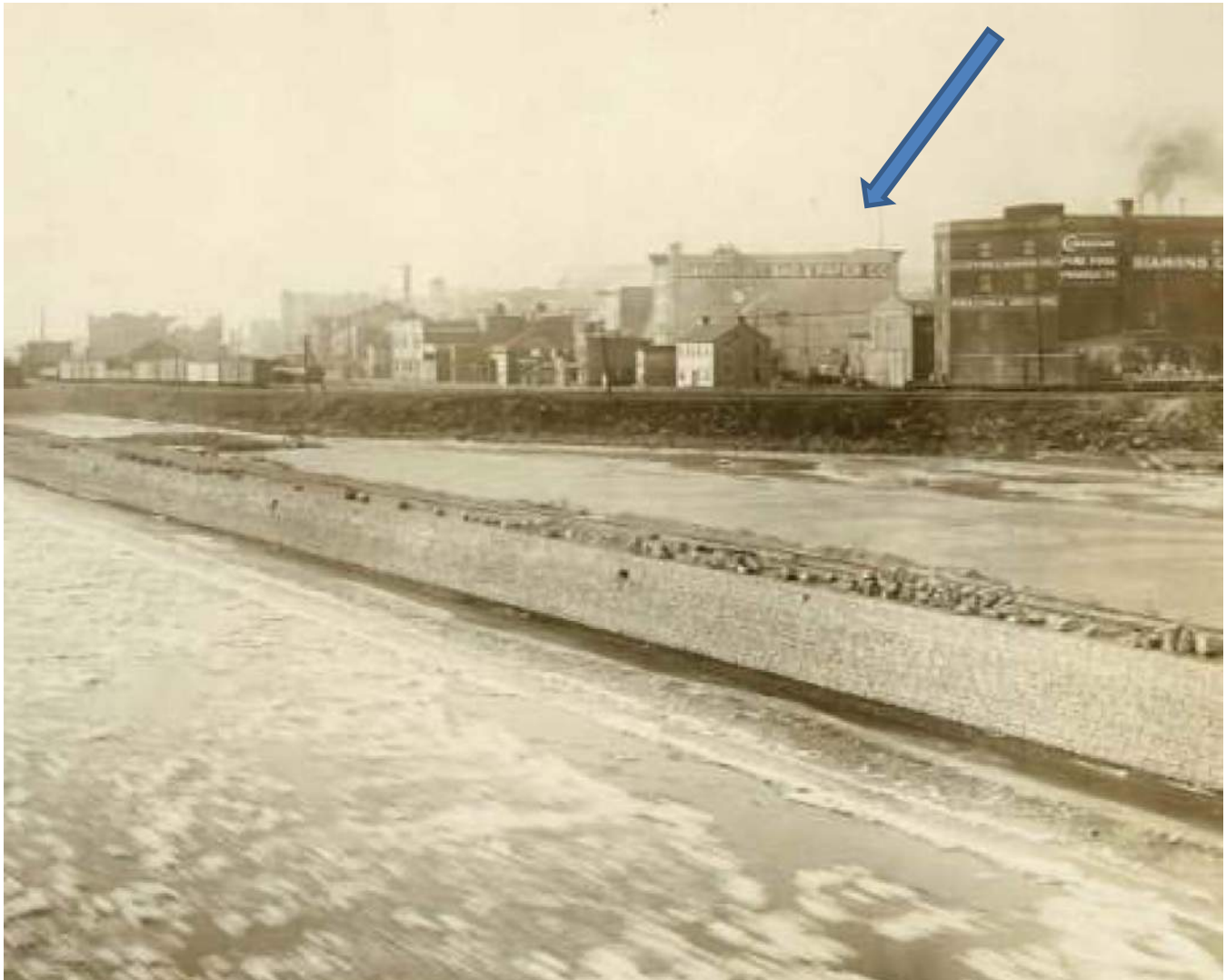
Photo was taken from Government Bridge, looking west ca. 1912. In the background some of the factories and prominent businesses that occupied Davenport's East End, including the Davenport Bag & Paper Company, are visible.
