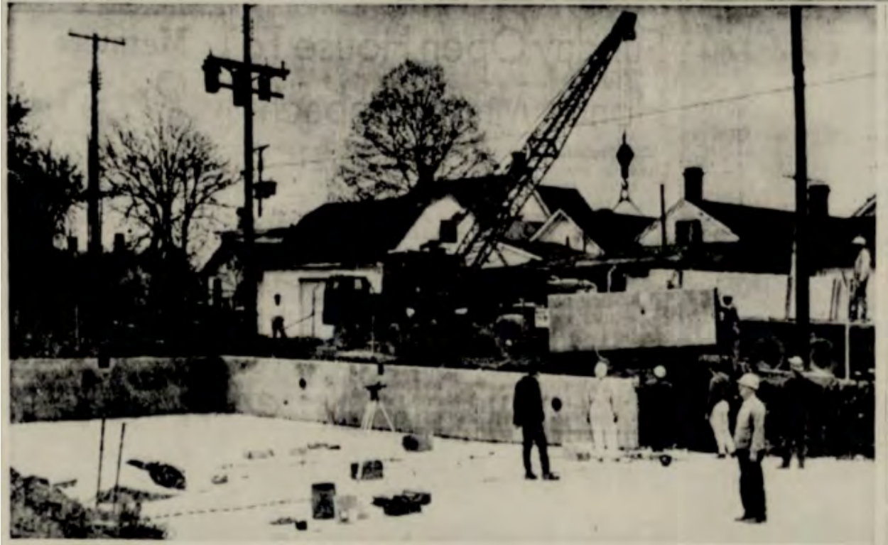
Figure 14: McKinley Pool under construction in April, 1967 ( Portsmouth Times ).
