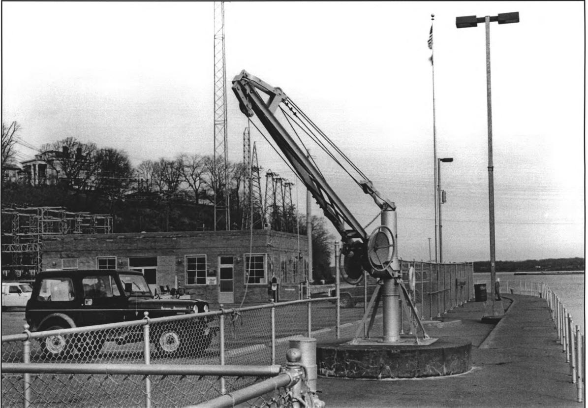
PHOTO 22. Upstream Land Wall Boat Davet on New Lock. Office and shop in the background. Incoming power transformer immediately to left of office and shop building. The other three boat davets on the new lock are identical to the one pictured here.
