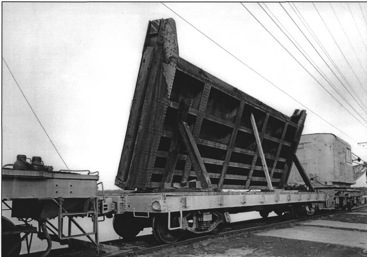
PHOTO 11. Flat Car Atop Dam Carrying Dam Gate.
