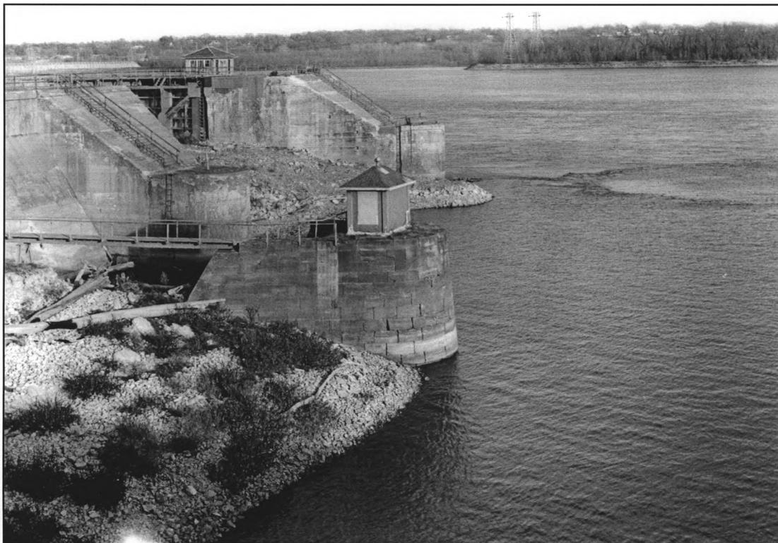
PHOTO 6. West Side of Des Moines Rapids Canal Bullnose. Stage recorder on top and depth recorder on west side installed before 1927. Downstream end of old lock in background. Note: old lock valve operating machinery shelter on the river wall of the old lock. Downstream side of rock retaining dike filling space in which miter gates would close visible. Earth berm in foreground lies between the new lock's river wall and the land wall of the dry dock.
