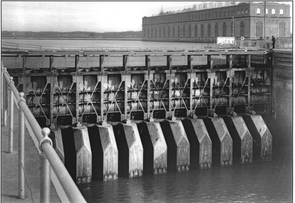
PHOTO 21. Upstream Vertical-lift Service Gate of New Lock, Downstream Side.
