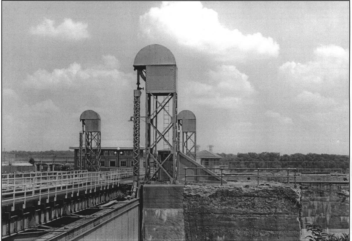
PHOTO 13. Three Pneumatic Hoist Towers. The one in the foreground operated the dry dock gate. The one in the left rear operated the emergency lock gate. The one in the right rear, the main upstream lock gate.
