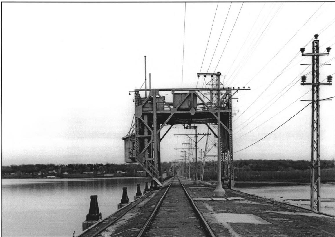
PHOTO 10. Traveling Gantry Crane Atop the Dam. Note large transmission towers visible behind the crane. The 22 smaller "phone pole scale" lattice towers on the dam are not important enough or large enough to be listed as individual components of the site. They are, in National Register terms, minor resources that do not contribute strongly to the property's historic character. The wires that run on these lattice towers only supply power for operating things on the dam.
