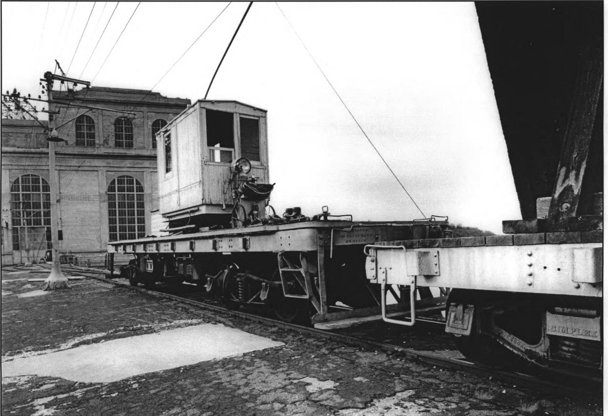
PHOTO 12. Electric-Powered Flat Car, with Top Floor of the Power Plant in Background.
