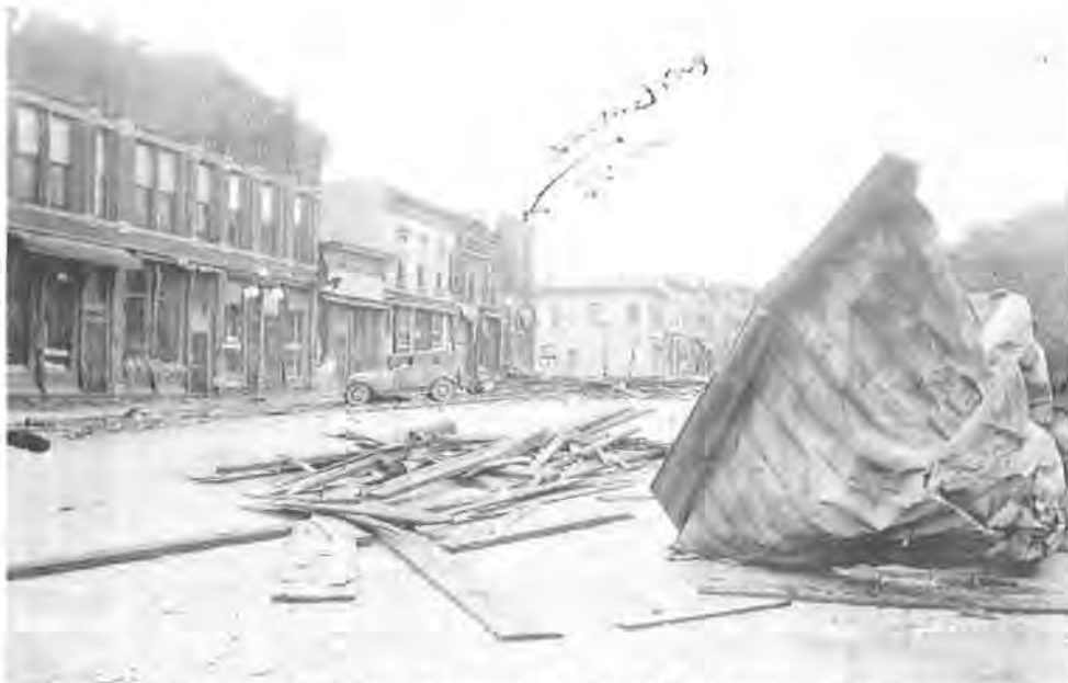
Figure 1 Storm damage, 1934. The crumpled heap of material in the right foreground is the pressed metal cornice from the Union Drug building noted in the background. From a newspaper clipping in the collection of Richard O. Woodard.
