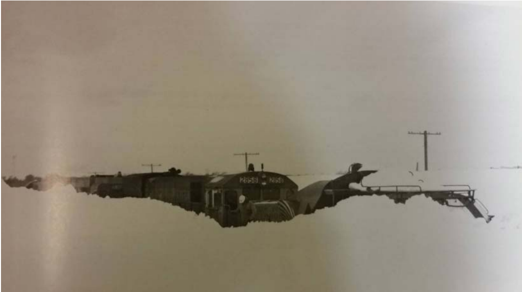
HP1 - UP Snow Plow No. 90013 being pulled into the clear on March 16, 1977 after derailing outside of Cheyenne Wells, Colorado. From James L. Ehernberger, "Engine Tender Snow Plows," The Streamliner . Volume 6, Number 3, p. 10; Union Pacific Historical Society, 1990.
