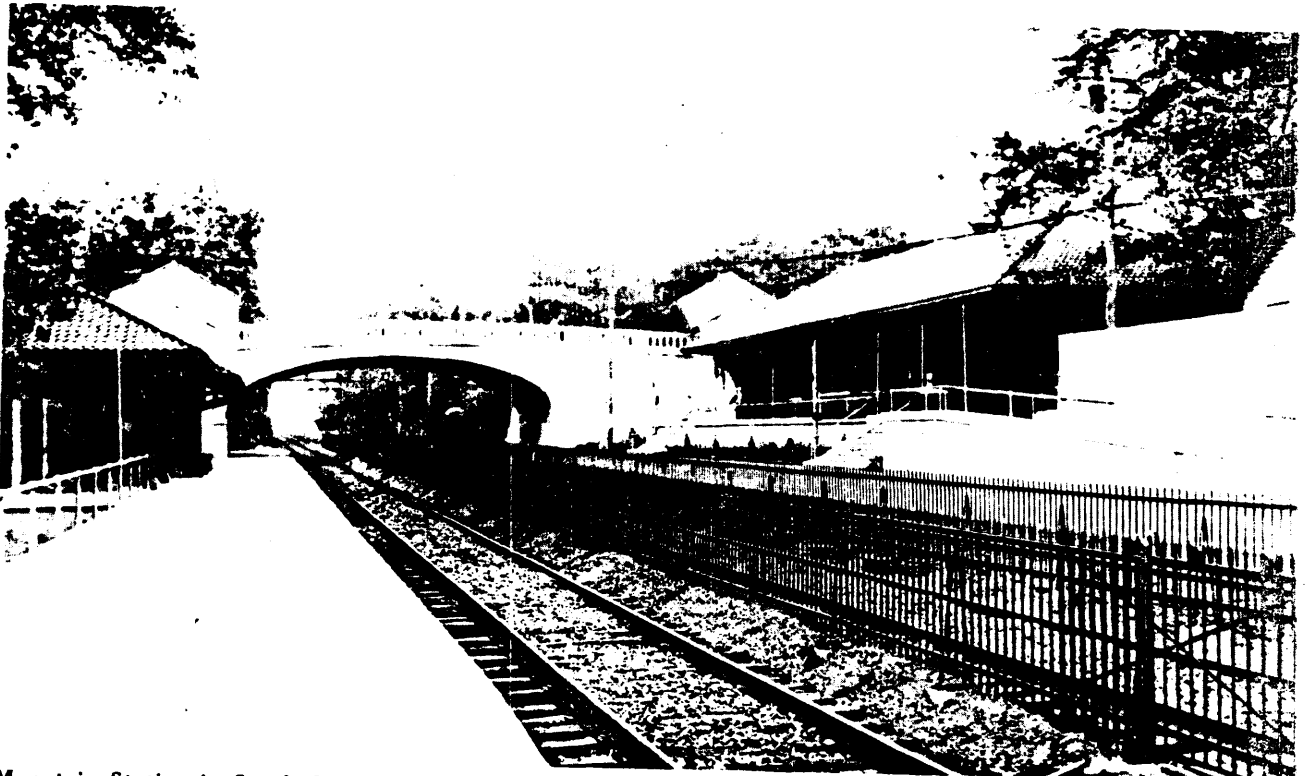
Mountain Station in South Orange was somewhat unique between Maplewood and Harrison. It was the only loc where the track elevation was not changed. In 1914 and 1915 Montrose Avenue was elevated over the tracks and new brick station constructed. At the same time the tracks were elevated at South Orange station.
