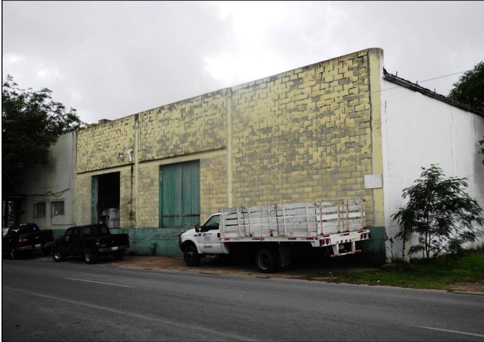
PHOTO 15: 454 E. Fronton Street (Resource 5), front/north and west elevations, facing south.
