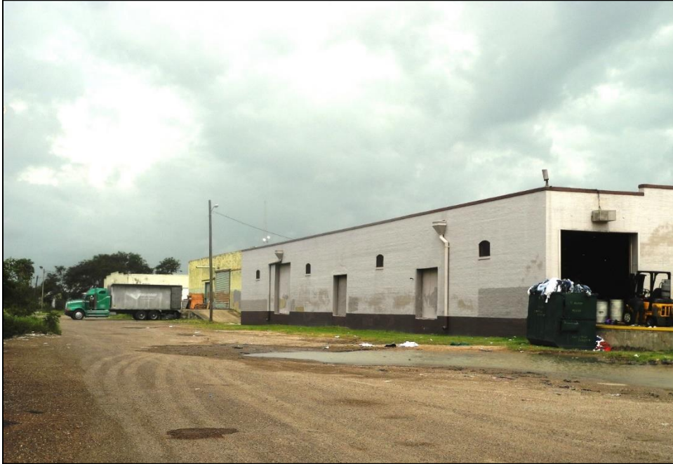
PHOTO 31: 504 E. Fronton Street (Resource 6), rear (freight line) elevations, facing north.
