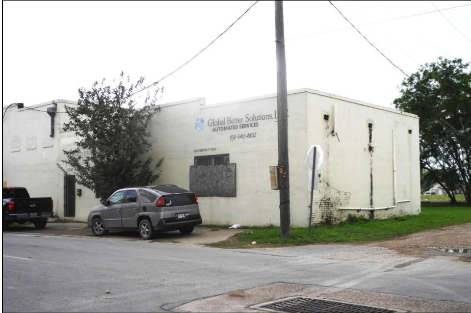
PHOTO 13: 430B E. Fronton Street (Resource 3), side and front/north elevations, facing south.
