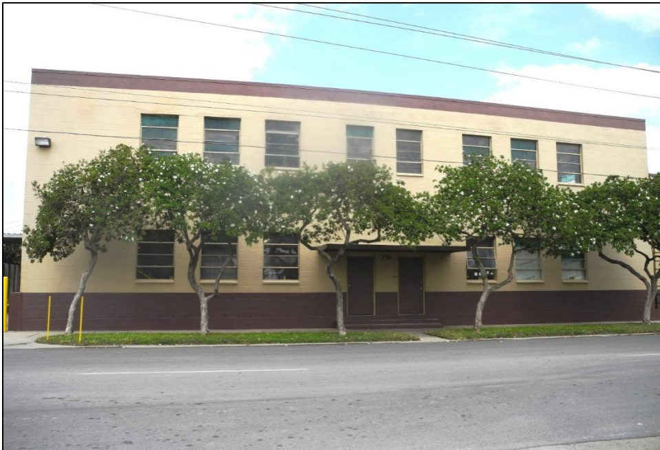
PHOTO 26: 739 E. Fronton Street (Resource 16), front/south elevation, facing northeast.
