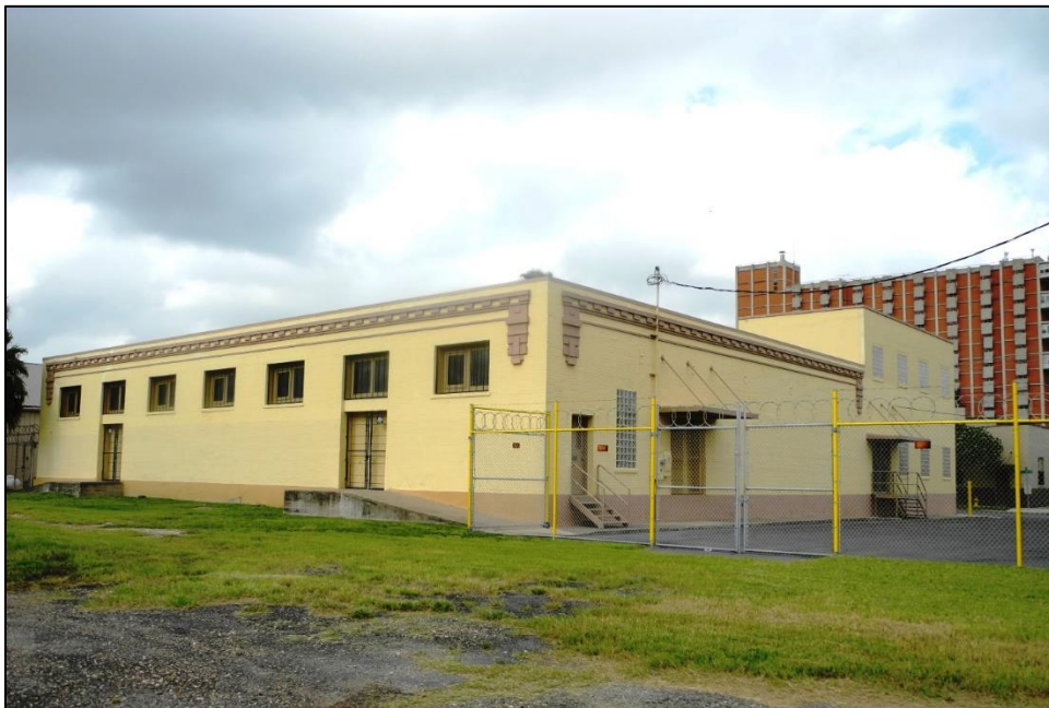
PHOTO 22: 730 E. Fronton Street (Resource 12), rear/south and east elevations, facing north.
