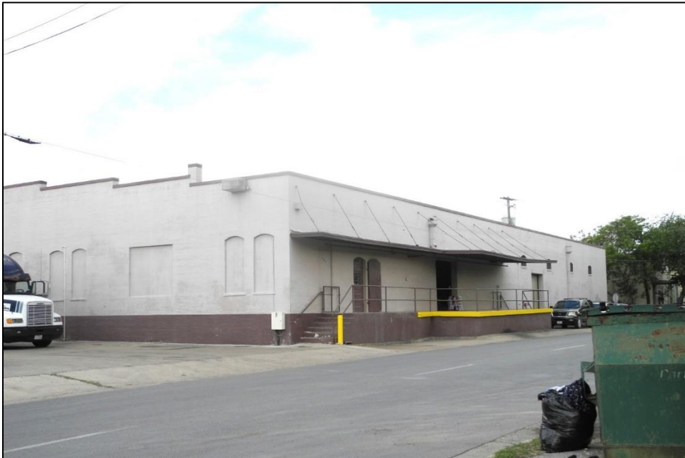
PHOTO 16: 504 E. Fronton Street (Resource 6), east and front/north elevations, facing west.
