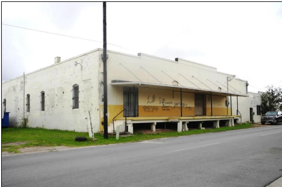
PHOTO 14: 430A E. Fronton Street (Resource 4), side and front/north elevations, facing west.
