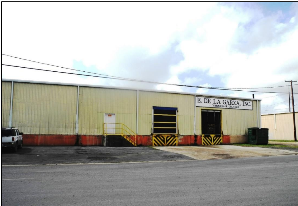
PHOTO 18: 600 block E. Fronton Street (Resource 8), front/north elevation, facing west.
