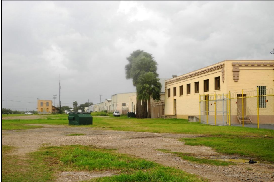
PHOTO 7: Rear (freight line) view along rear, 400-700 blocks E. Fronton, facing north/northwest.
