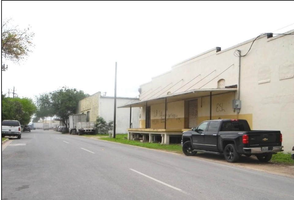
PHOTO 5: 400-500 blocks E. Fronton Street (Resources 4 and 5 showing right to left), front/north elevations, facing south.
