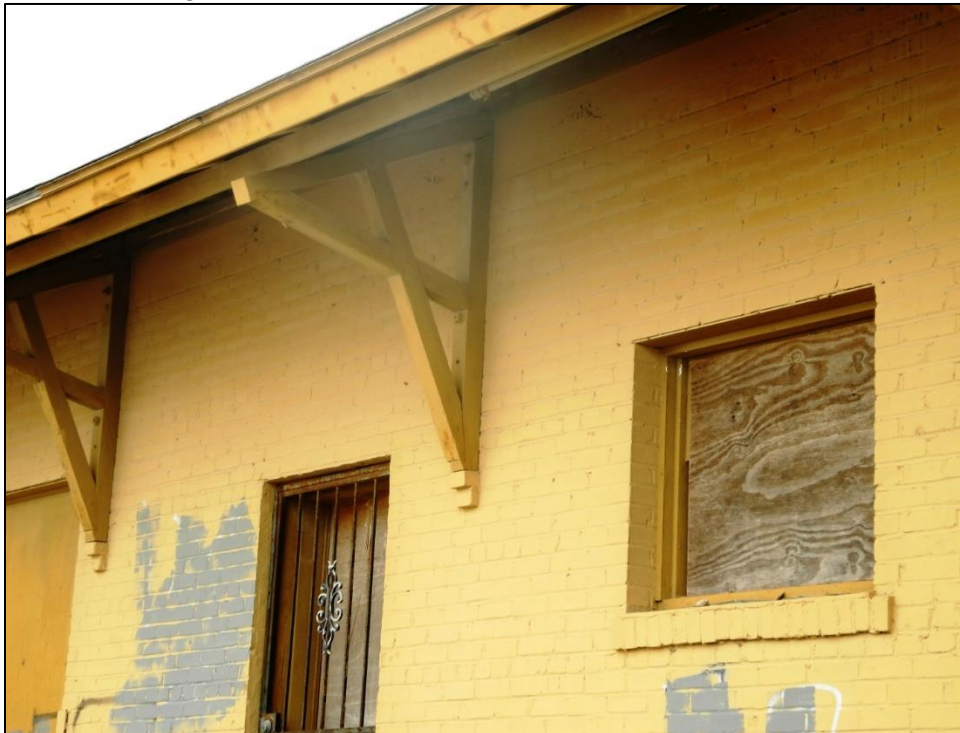
PHOTO 28: Bracket and brickwork detail, St. Louis, Brownsville & Mexico Railway Co. Depot, south elevation, facing northwest.
