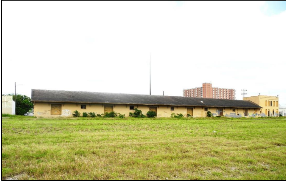
PHOTO 1: St. Louis, Brownsville & Mexico Railway Co. Freight Depot (left) and Depot Office (right), (Resources 1 and 2), front/south elevations, facing north/northeast.
