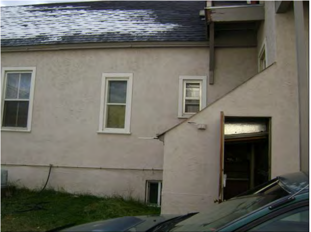
MT_LewisAndClark_Lyman-NeelResidence_0011: Lyman-Neel Residence. One-Story Addition, North Elevation, looking south.
