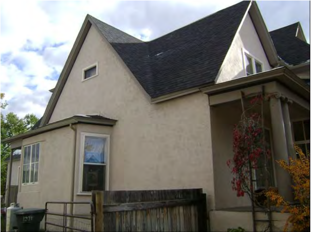
MT_LewisAndClark_Lyman-NeelResidence_0007: Lyman-Neel Residence. Two-Story Portion, North Elevation, looking southeast.
