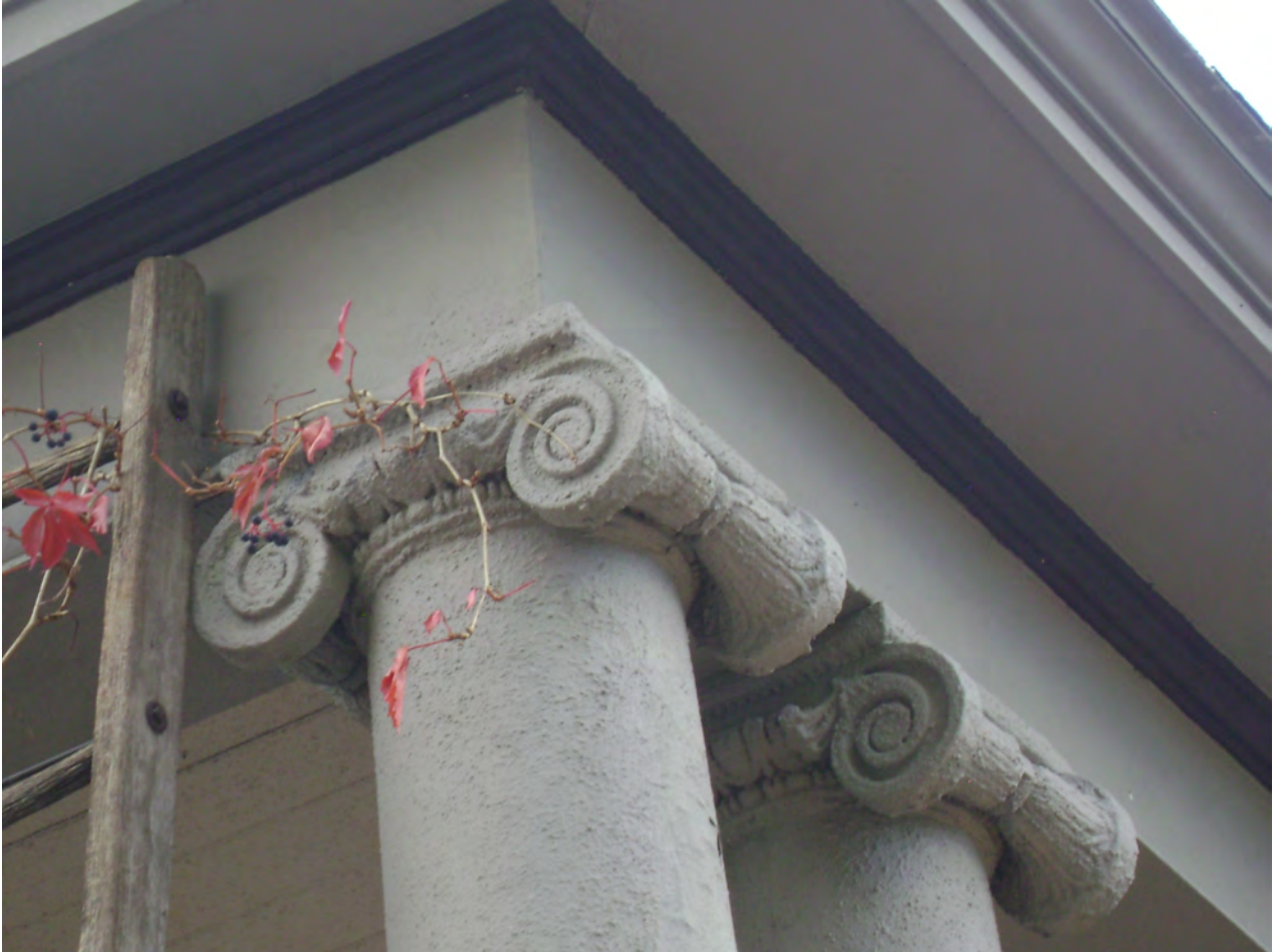
MT_LewisAndClark_Lyman-NeelResidence_0003: Lyman-Neel Residence. West Elevation NW corner, looking SE. Ionic column detail.
