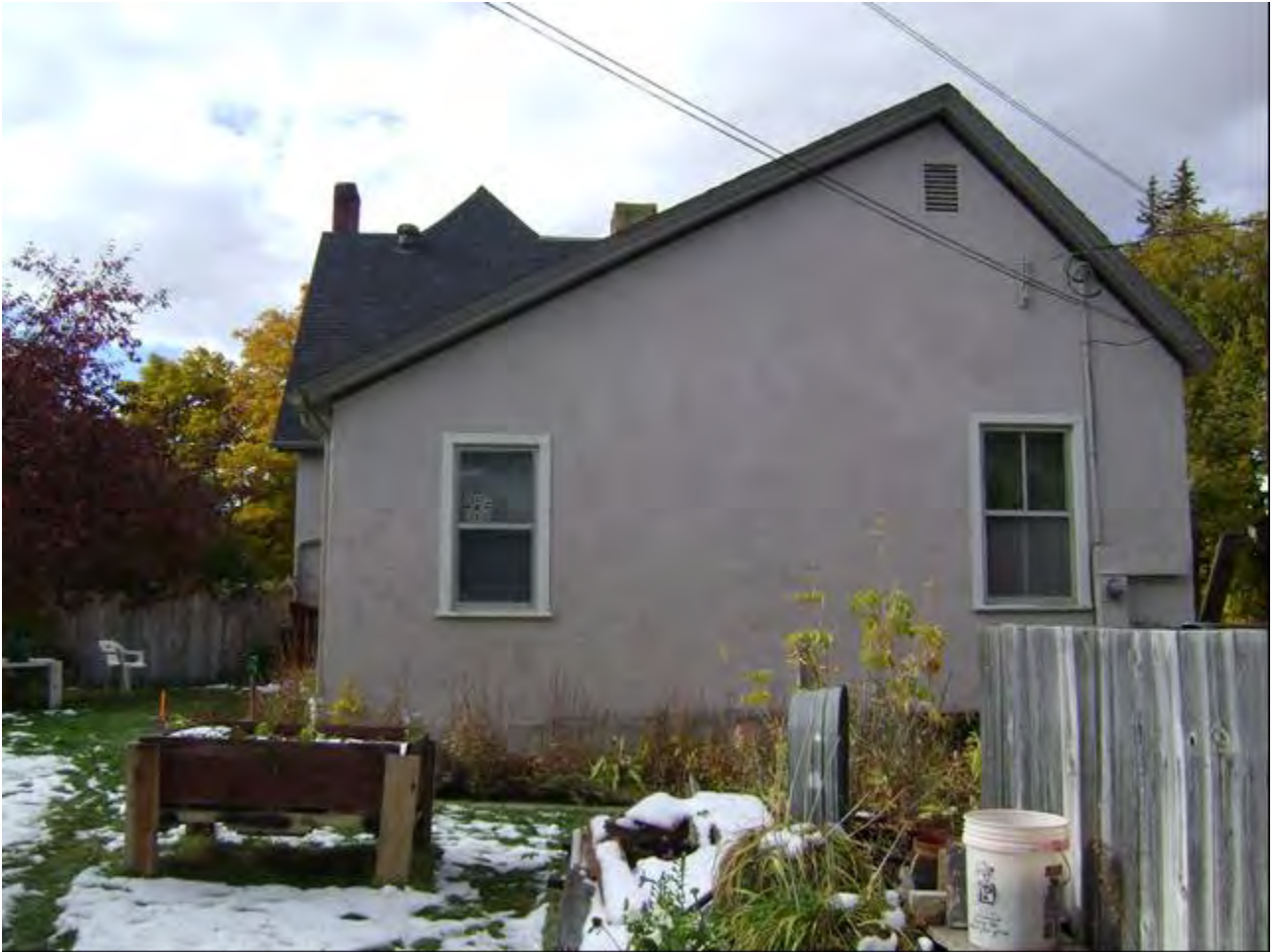
MT_LewisAndClark_Lyman-NeelResidence_0010: Lyman-Neel Residence. One-Story Addition, East Elevation, looking west.
