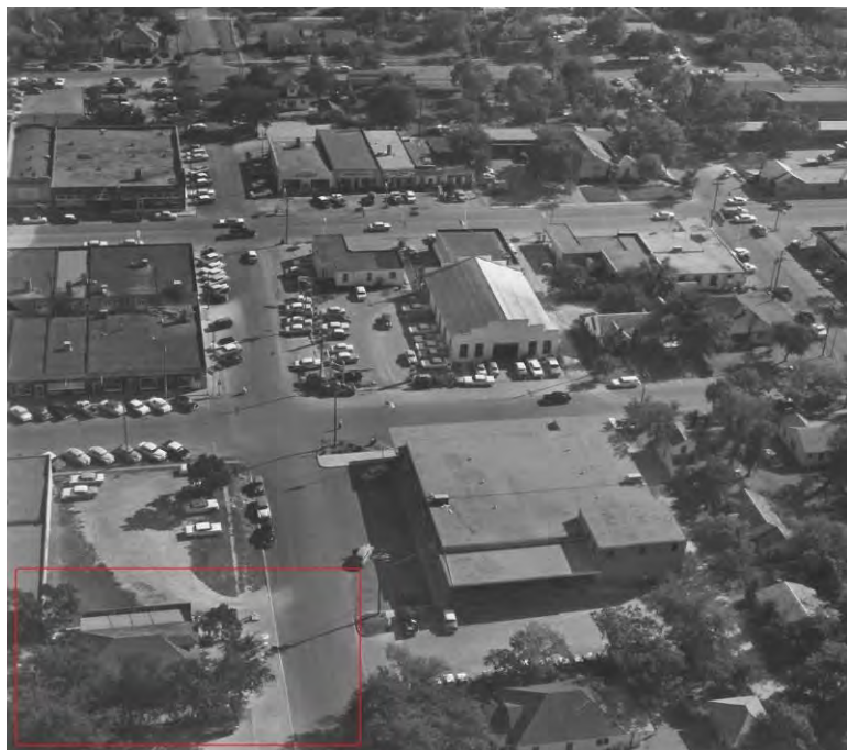
Figure 8: View looking southwest toward 212 N. 7 th Street, marked in red. Note the shed constructed the length of the south elevation, c 1958. Courtesy of the Garland Landmark Society.
