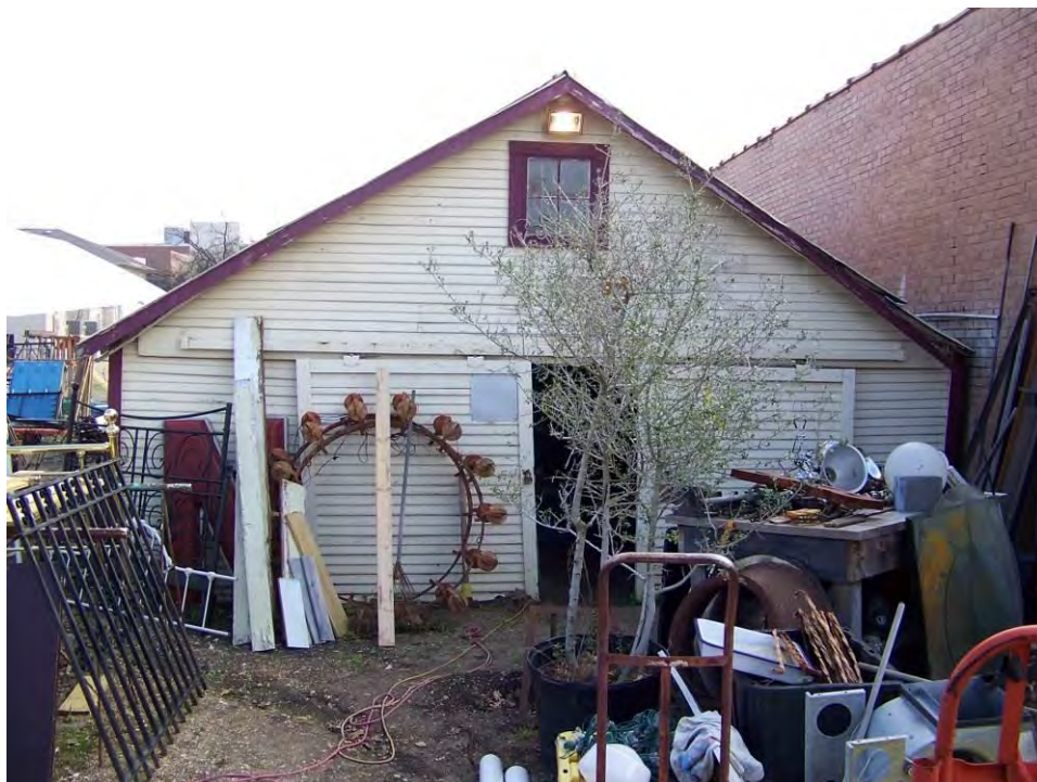
Photo 5: View east from backyard of west elevation of garage. Camera facing east.
