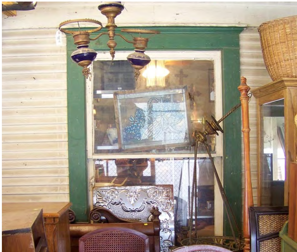
Photo 11: View of original window, trim and wood siding under the south shed. Camera facing north.
