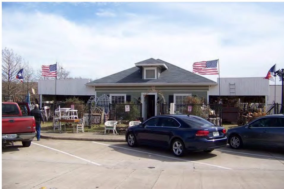
Photo 1: View east from 7 th Street at front/west elevation of house. Camera facing east.
