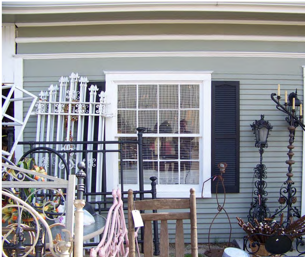
Photo 13: Note the trim in the cornice is similar to trim in Figure - 4. This is one of the few clues that Figure - 4 might be the original porch. Camera facing east.
