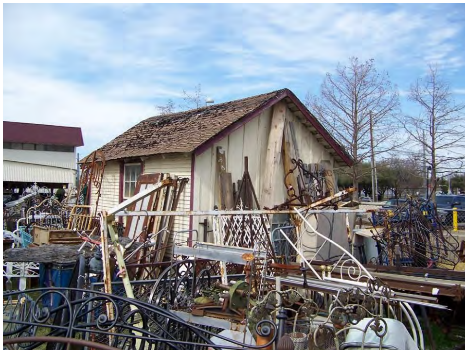
Photo 8: View of bedroom structure. Camera facing northwest.
