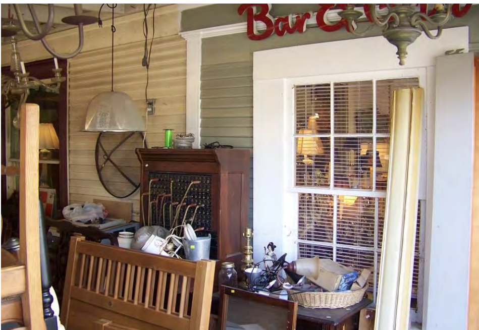
Photo 10: View of north porch enclosure wall painted green paint. The original window installed at this location at time of enclosure was used to replace deteriorated front window. This window is from a salvage yard and selected because it matched original. Camera facing southeast.
