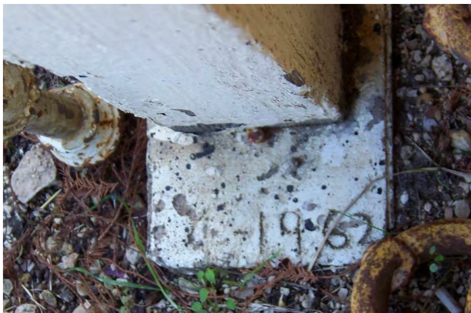
Photo 12: View inscribed concrete footing at the northeast column of shed.
