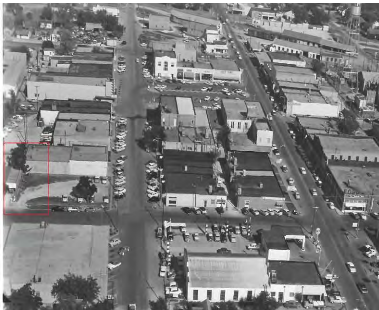
Figure 9: View looking east toward downtown, 212 N. 7 th Street marked in red at the edge of photograph. Note the shed constructed on the south elevation, c 1958. Courtesy of the Garland Landmark Society.
