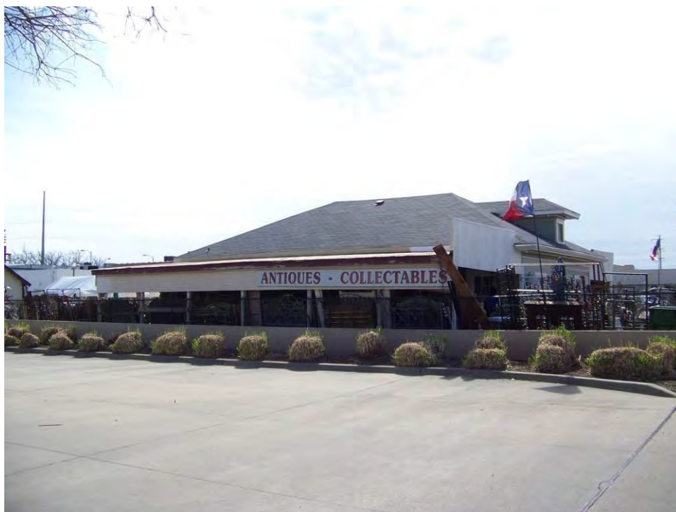
Photo 4: View southeast from 7 th Street sidewalk of north elevation of house. Camera facing southeast.
