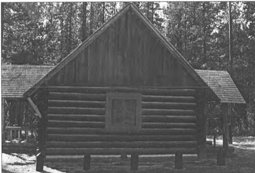
4 of 20: Exterior view, north facade View to south.
