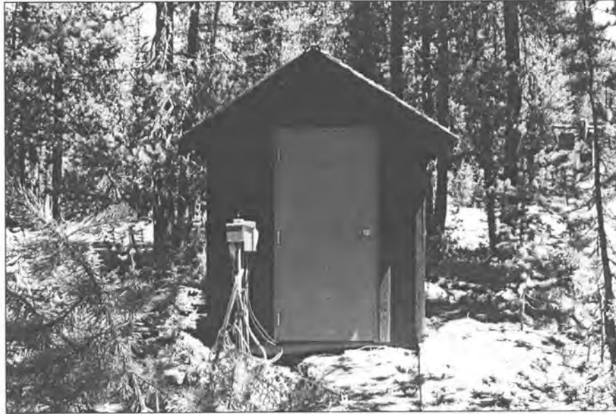
19 of 20: Exterior view, pump house.
