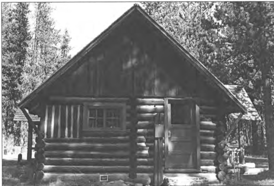
5 of 20: Exterior view, south facade. View to north.
