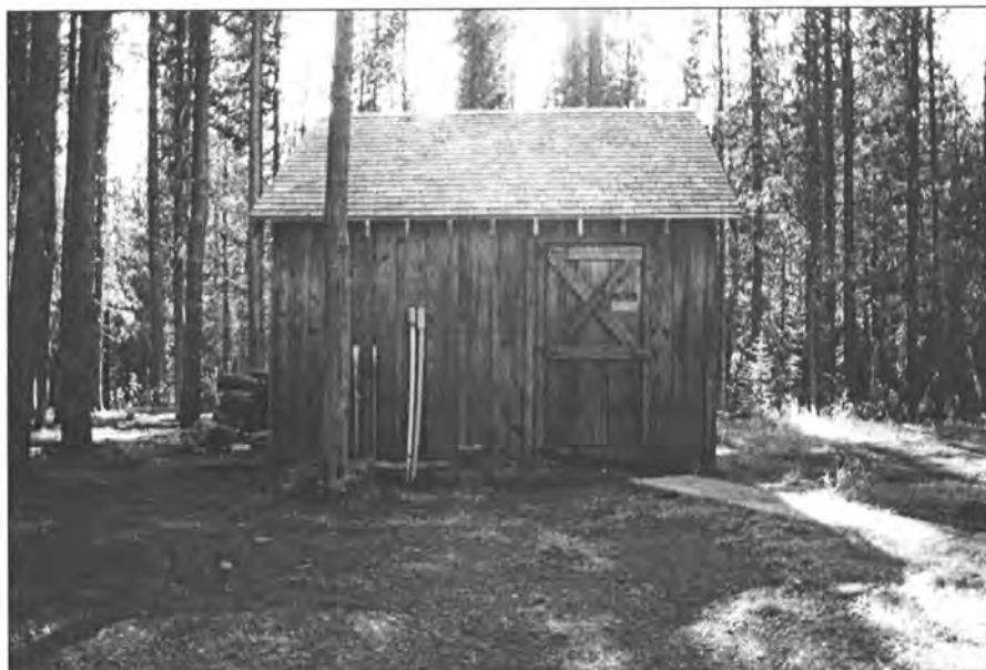
6 of 20: Exterior view, north facade, utility building. View to south.
