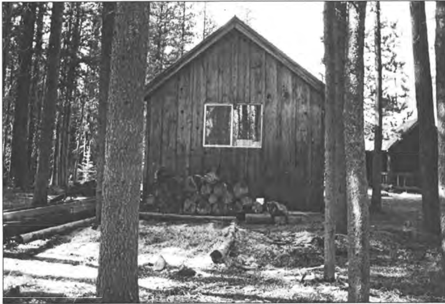
7 of 20: Exterior view, East facade, utility building. View to west.
