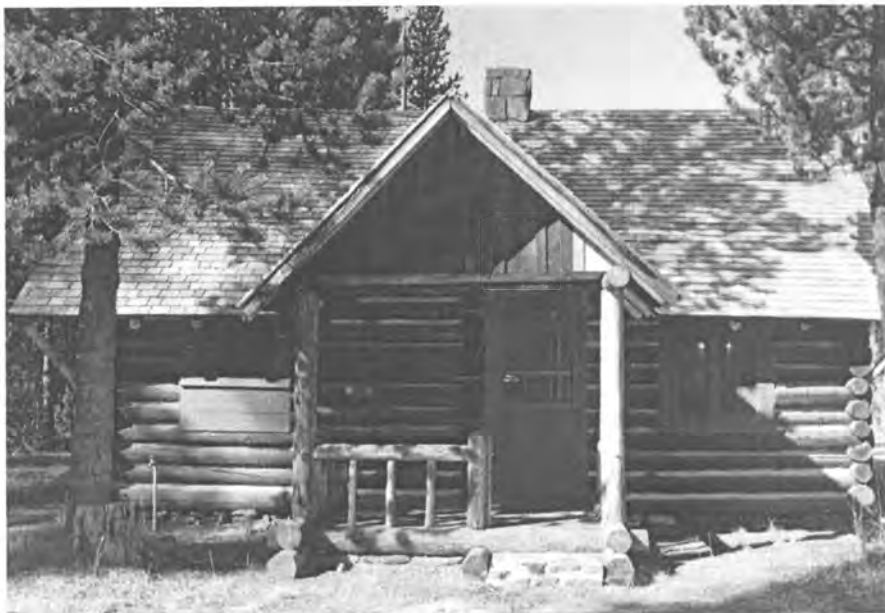
3 of 20: Exterior view, east (rear) façade. View to west.
