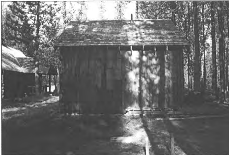
8 of 20: Exterior view, south facade, utility building. View to north.
