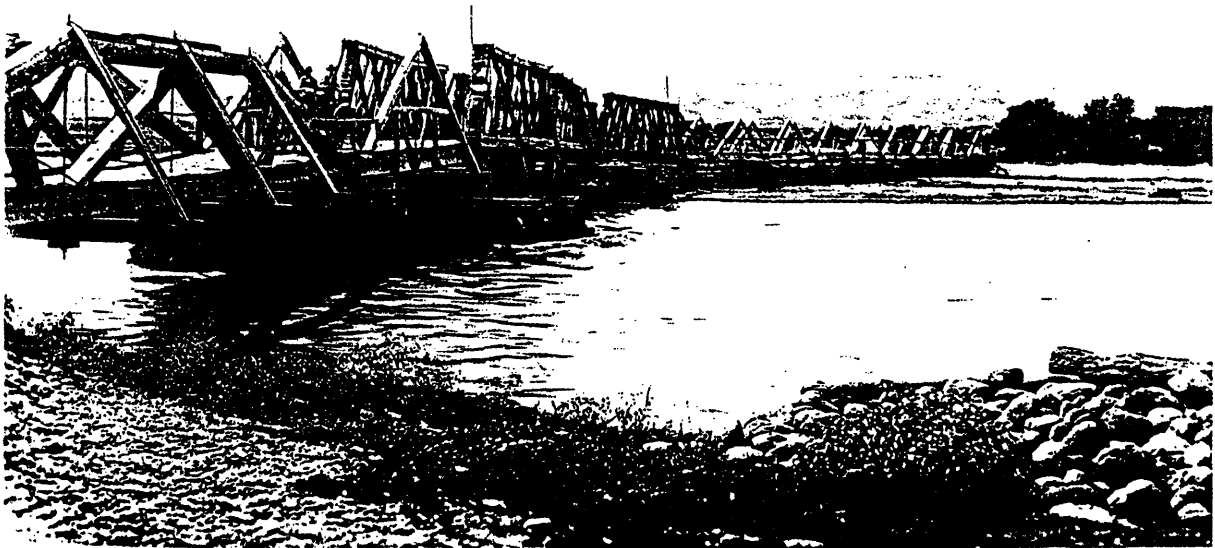
Timber Truss Across the Río Grande at Espanola About 1912. (Photograph Courtesy of the Museum of New Mexico, Negative No. 61684)
