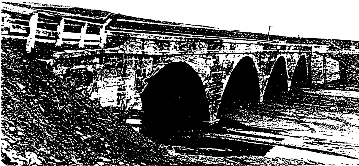
Canadian River Bridge near Springer. Completed prior to 1916, this bridge was typical of the concrete arch construction used at several locations in the state. (Highway Department Bridge Files, Inactive)
