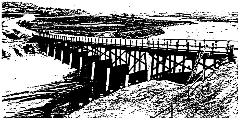
Revuelto Creek Bridge East of Tucum- cari. This bridge was completed on US 66 in 1931 using treated tim- ber construction. ( High- way Department Bridge Files , Inactive)
