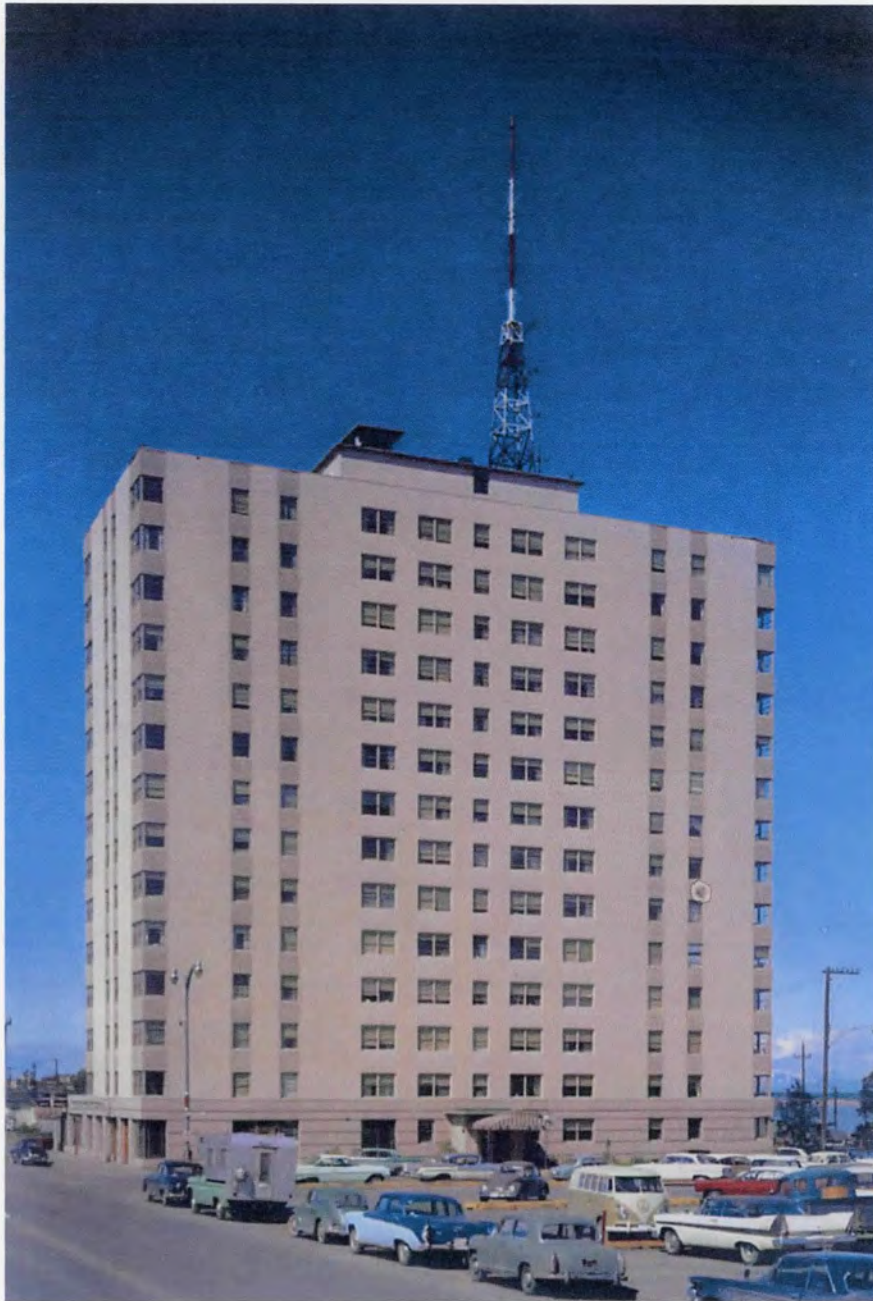
McKinley Tower Apartments, 1963 View of east elevation, facing northwest from across 4 th Avenue (Credit: Anchorage Museum Archives, 'Ektacolor negative, McKinley Apts.')
