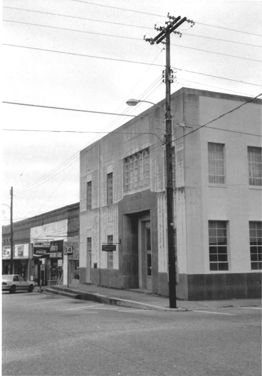
2. BARNETT BLVD. LOOKING SE
