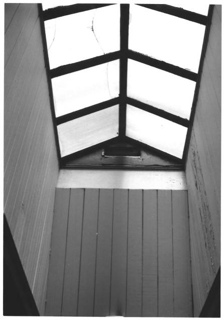
Skylight in center of second floor of store building is original, and made of wire glass in metal frames. Looking west
