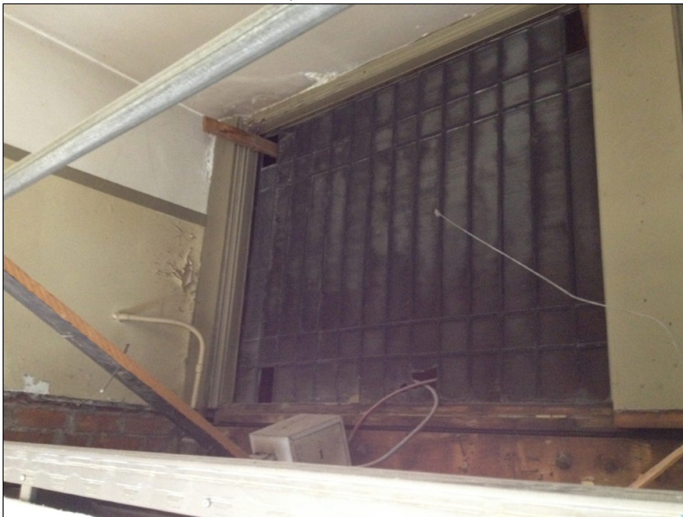
Detail of transom covered by pea stone soffit on facade and drop ceiling on interior of first floor (source: Aharonian & Associates Inc. 2017).
