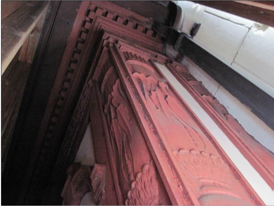
Detail photograph of the stamped sheet metal storefront beneath the pea stone soffit on the facade (Source: Aharonian & Associates Inc. 2017).
