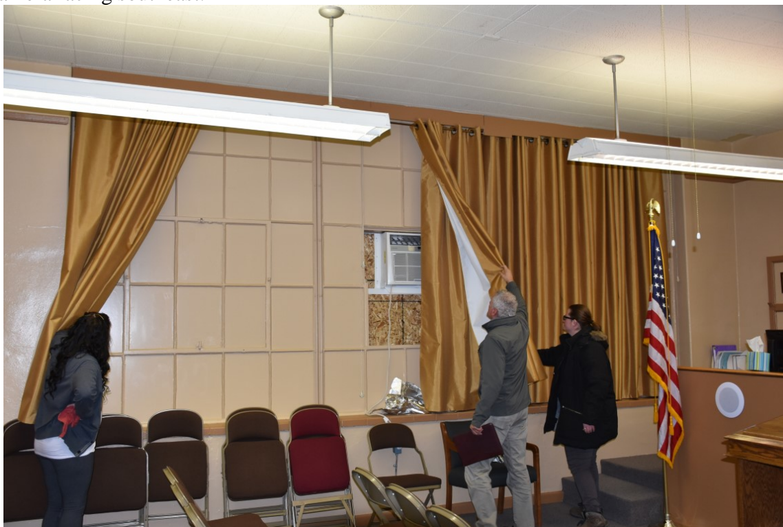
10 of 16. Interior view of southeast classroom showing original painted-over window. Camera facing southeast.
