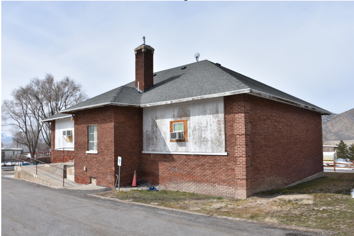
3 of 16. North and east elevations. Camera facing southwest.
