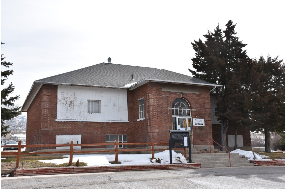
2 of 16. West and north elevations. Camera facing south.
