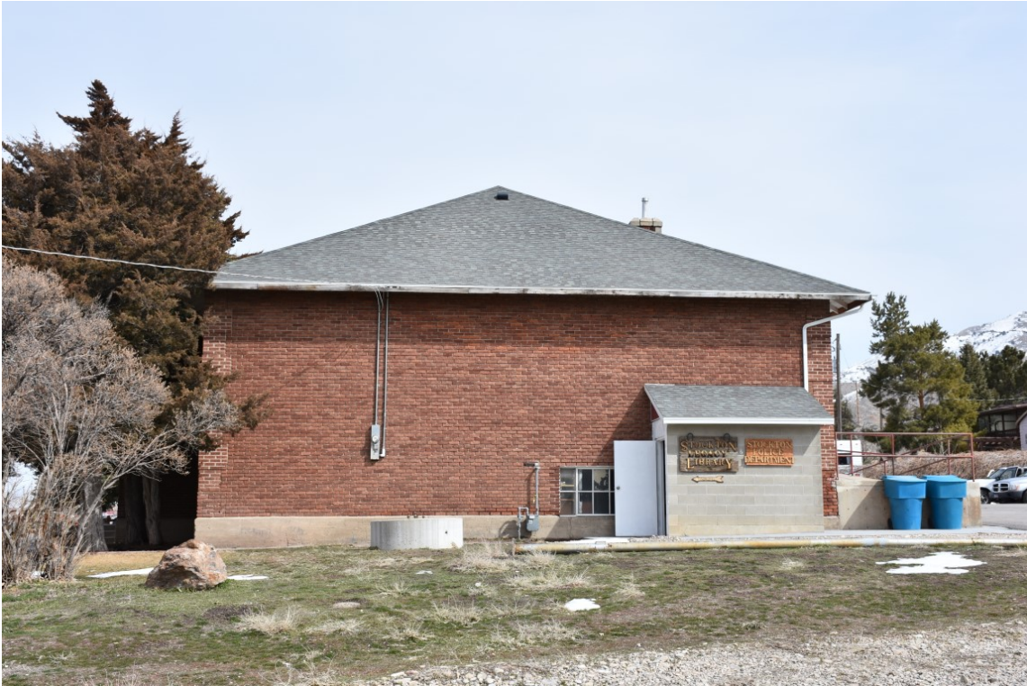
6 of 16. South elevation. Camera facing northeast.
