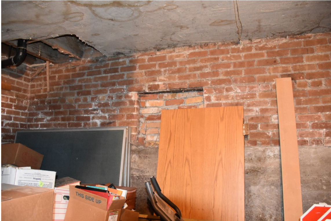
15 of 16. Interior of basement in unfinished north room. Camera facing northeast.
