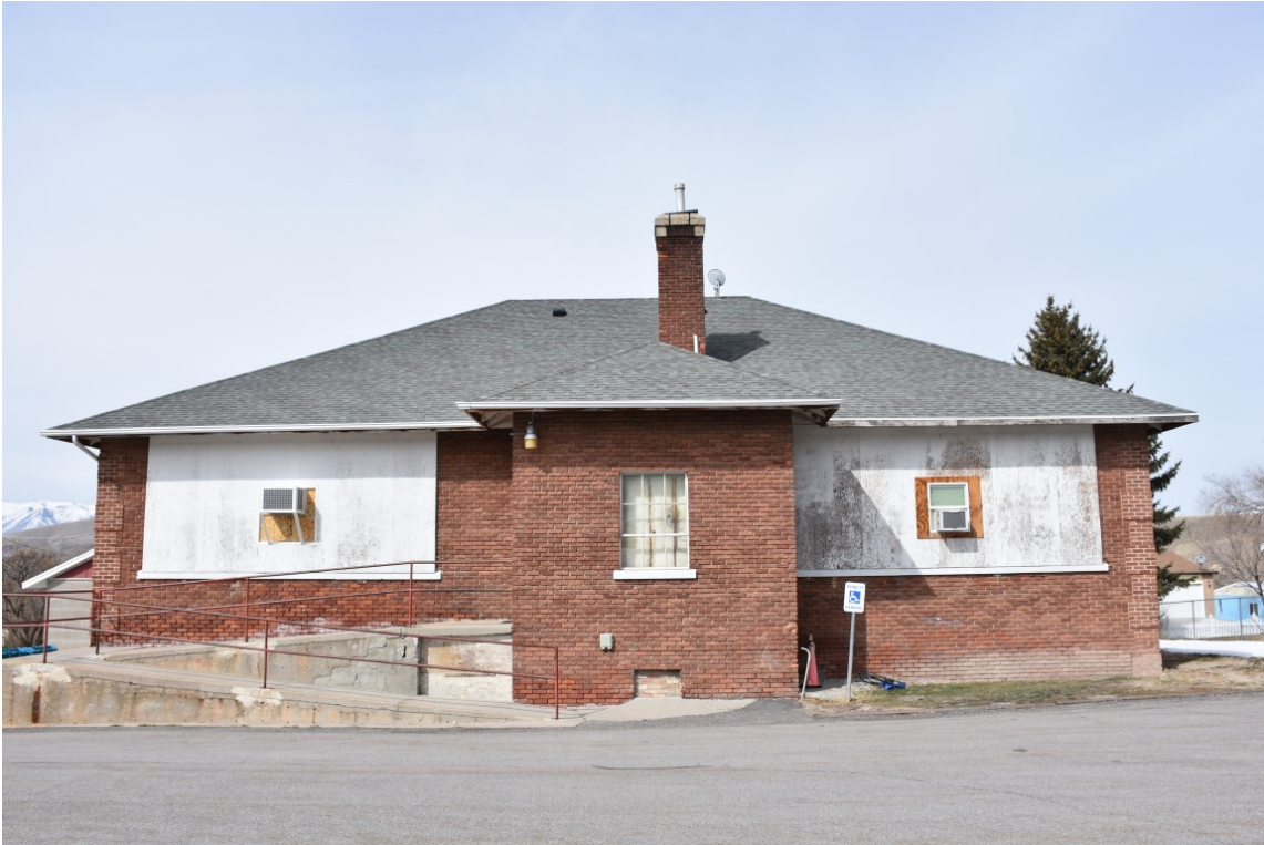
4 of 16. East elevation. Camera facing northwest.
