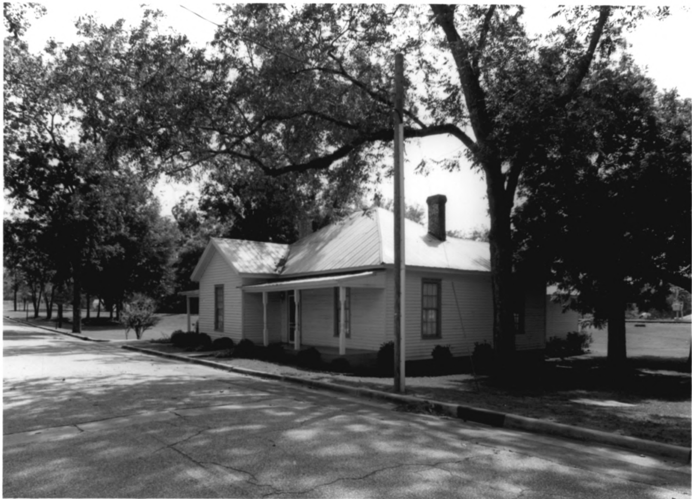
ALFRED AND JANE ABLES HOUSE BUENA VISTA, MARION COUNTY, GEORGIA PHOTOGRAPH 1 OF 12
