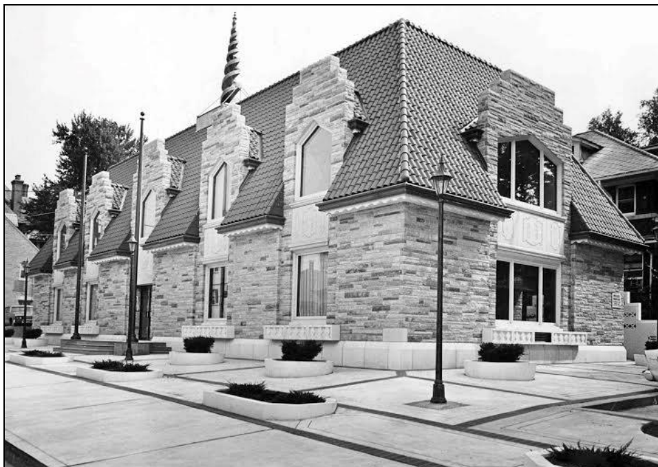
Figure 2: Newspaper photograph of the Danish Brotherhood building, 1966. Note the single-light, fixed sashes in the windows. From the Omaha World-Herald archives.
