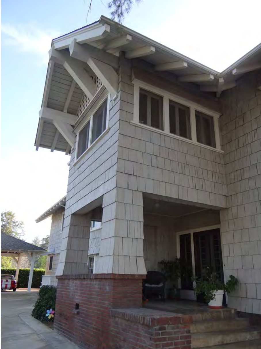
Photo 6. Back porch with square columns and sleeping porch. Camera facing south.
