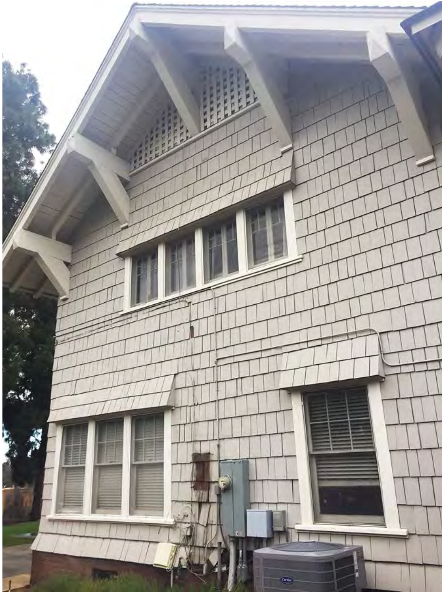
Photo 5. South east elevation. Camera facing west..
