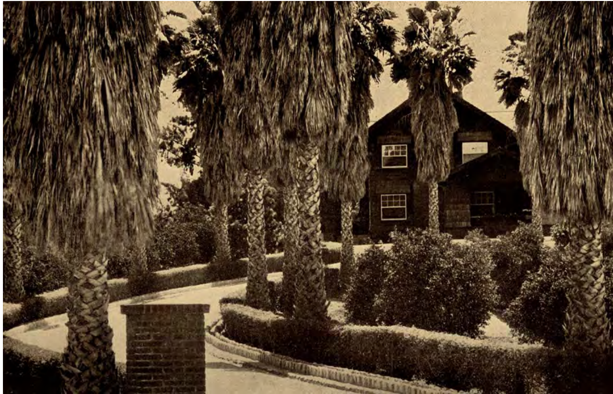
Figure 7. Original driveway and northwest elevation (McDaniel, 1927)
