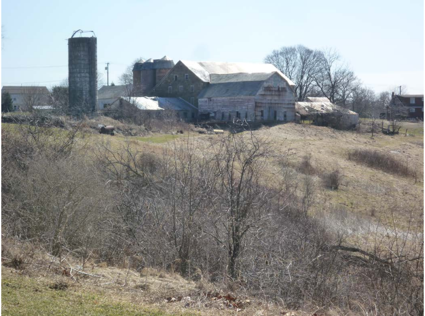
Figure 1: Looking East from the Harmony Mennonite Meetinghouse and Cemetery; former Shantz (Shontz) farm; stone barn c. 1835. Beyond this farm is a 1990's era group of tract homes illustrating the suburbanization of the area.
