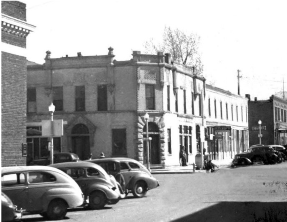
HP 29. 1940 view south on Pikes Peak, 100 E. Main Street (5FN.2280) center, edge of 101-103 E. Main Street (5FN.2281) visible at right. Photo courtesy of Florence Archives.
