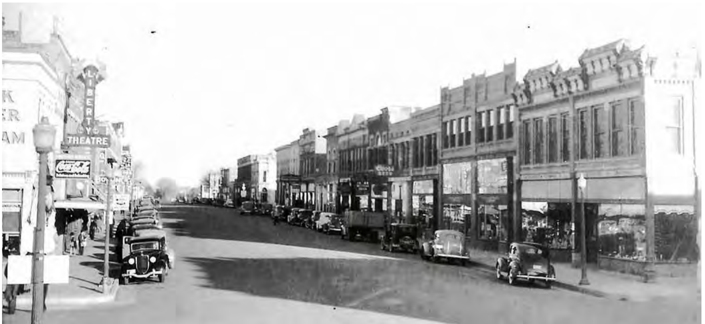
HP 27. Main Street view east, 1937. From right to left, 129-131 W. Main Street (5FN.2315), 125-127 W. Main Street (5FN.2313), 123 W. Main Street (5FN.2311), 121 W. Main Street (5FN.2309), etc. Photo courtesy of Florence Historical Archive.
