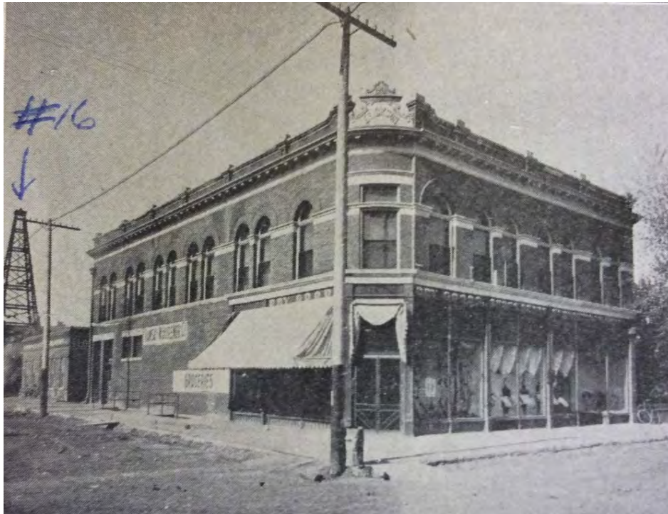
HP 8. 100 E. Main Street (5FN.622), Hotel Florence, 1906, with Oil Derrick 16 highlighted. Photo courtesy Florence and its Environs, Florence Historical Archive.
