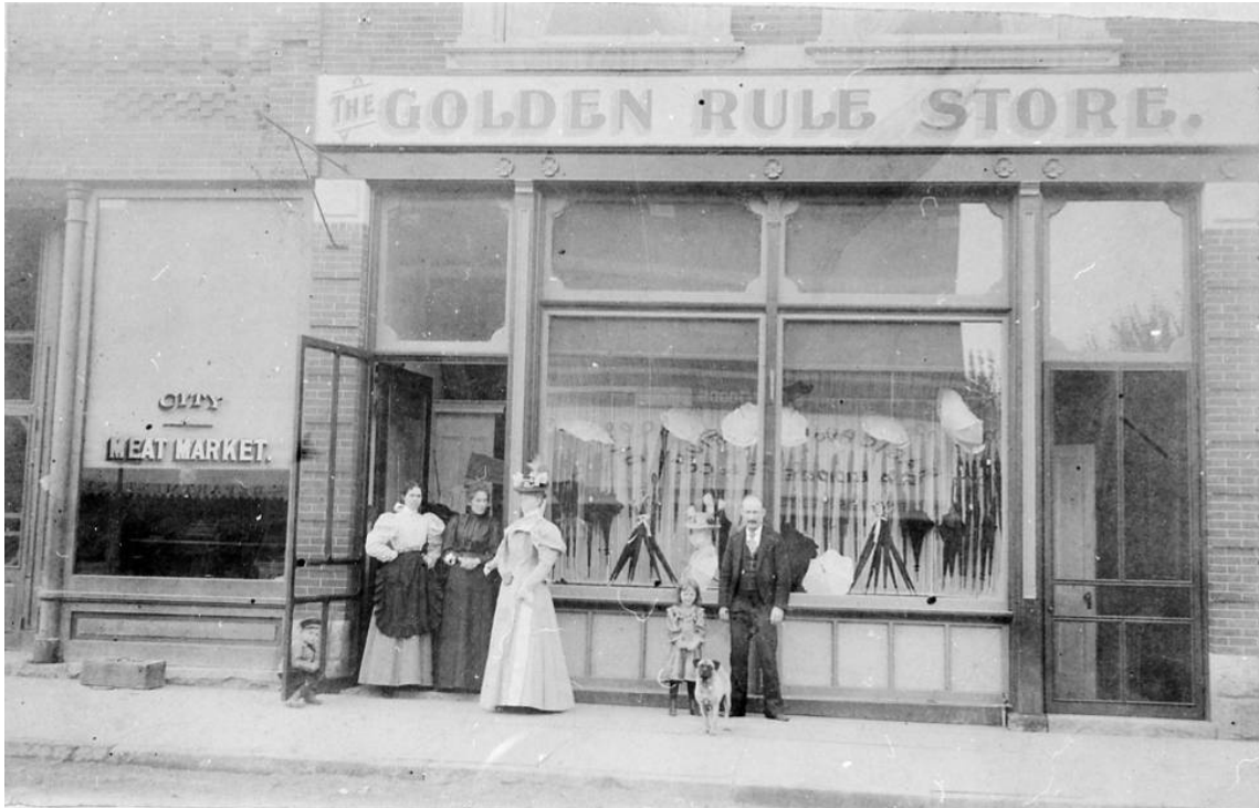
HP 13. 113 W. Main Street (5FN.2305) Golden Rule Store, and edge of 111 W. Main Street (5FN.2303) City Meat Market visible at left, photo 1906. Photo courtesy Florence Historical Archive.
