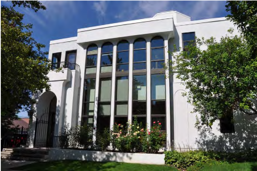
Photograph 6 of 10 East elevation detail, Western General Agency Building. Camera facing west.
