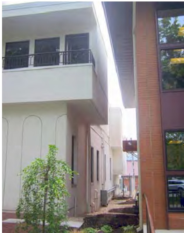
Photograph 4 of 10 West elevation, Western General Agency Building. Camera facing south.
