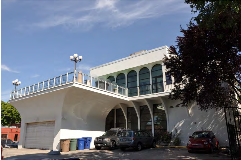
Photograph 3 of 10 South elevation, Western General Agency Building. Camera facing northwest.
