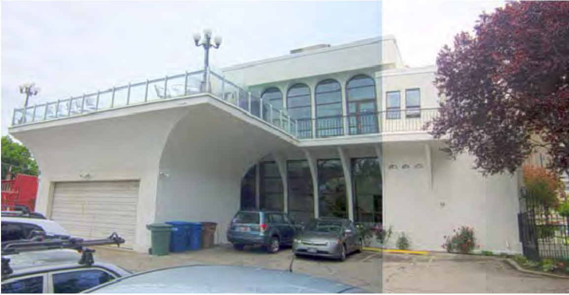
Photograph 3 of 10 South elevation, Western General Agency Building. Camera facing northwest.
