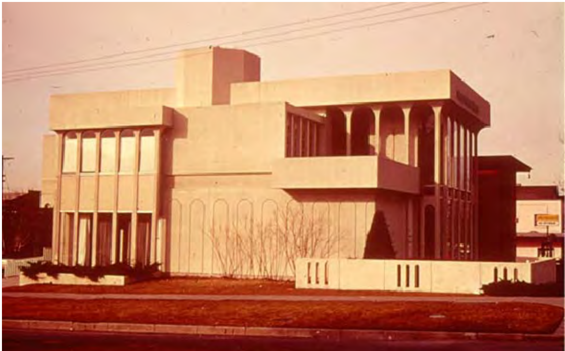
Figure 2 c. 1971 photograph of the Western General Agency from the east.
