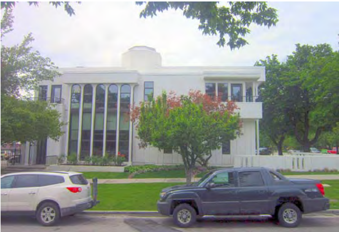
Photograph 2 of 10 East elevation, Western General Agency Building. Camera facing west.
