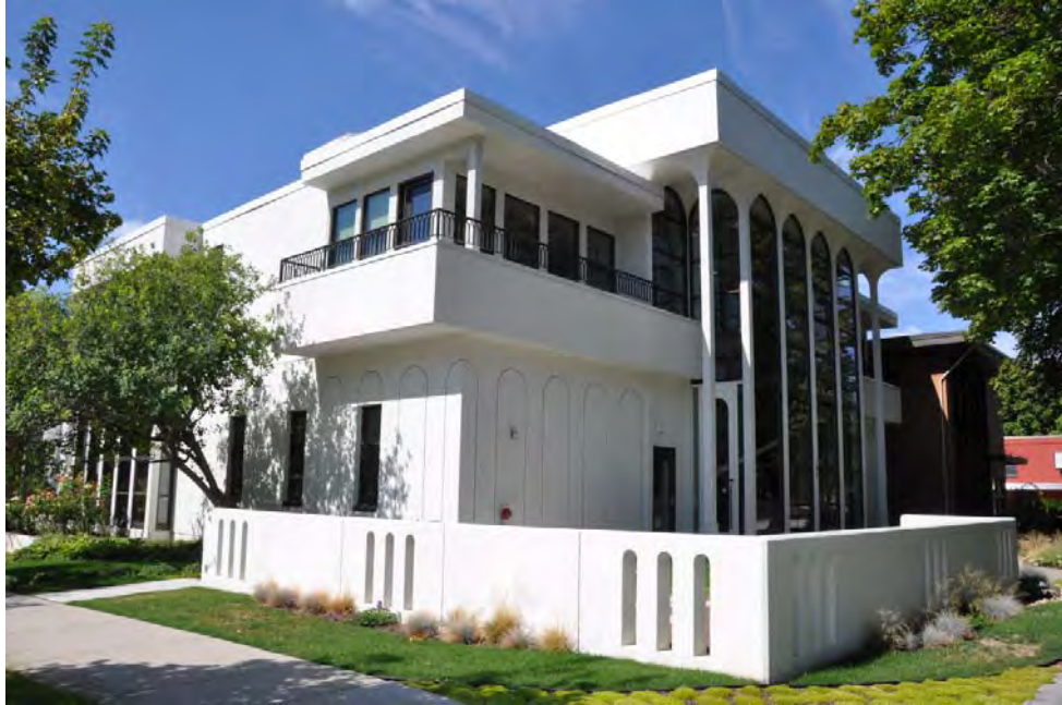
Photograph 5 of 10 North and East elevations, Western General Agency Building. Camera facing southwest.
