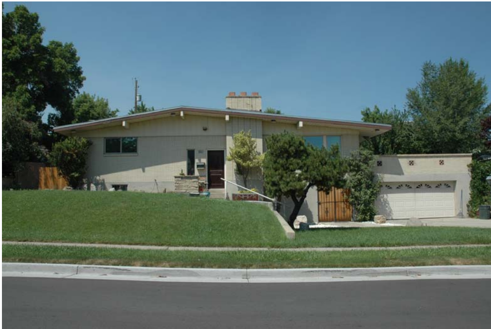
Photograph 41 of 44 View of 5560 S. 235 East. Camera facing west.
