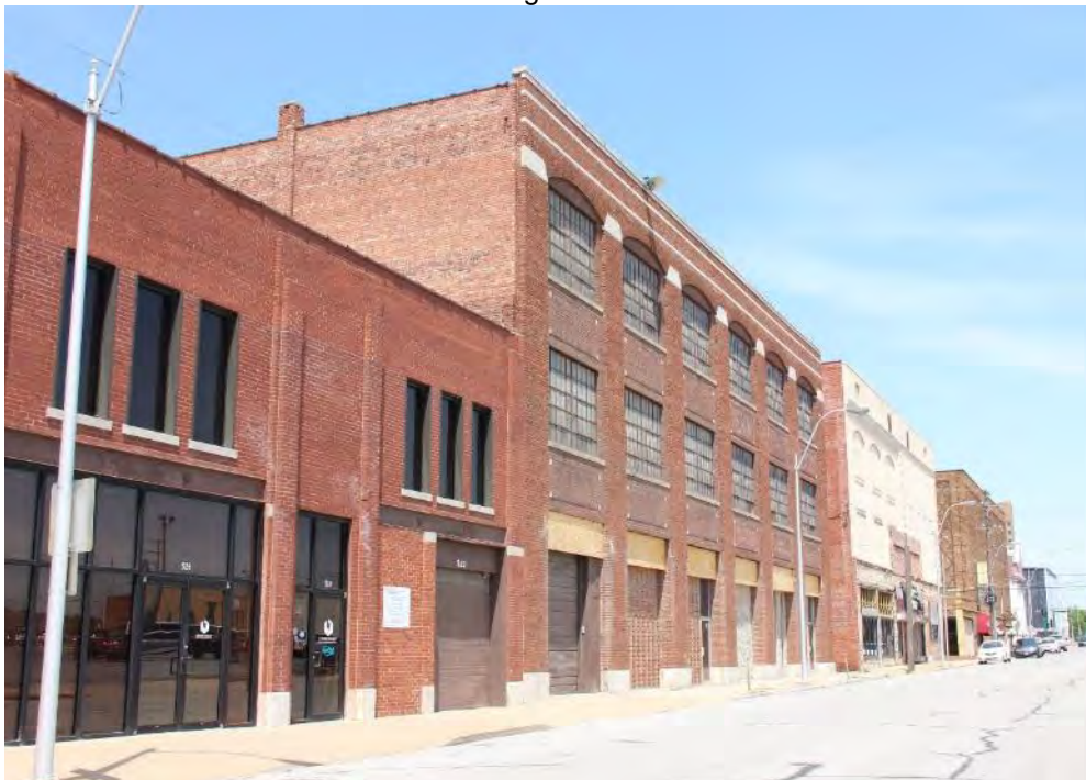
4 of 26: Southeast corner. Camera facing northwest.
