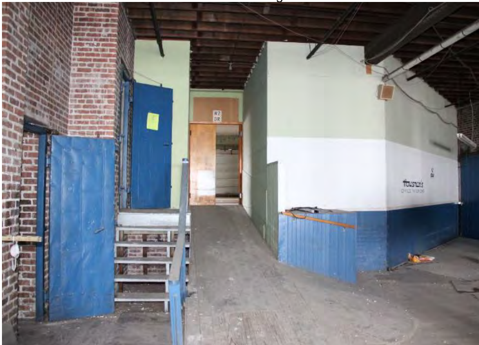
20 of 26: Second floor north side. Camera facing west.
