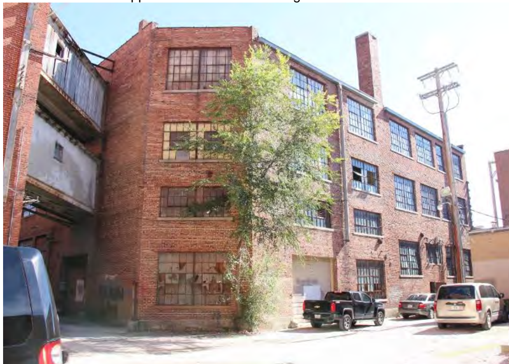
6 of 26: Northwest clipped corner. Camera facing southeast.
