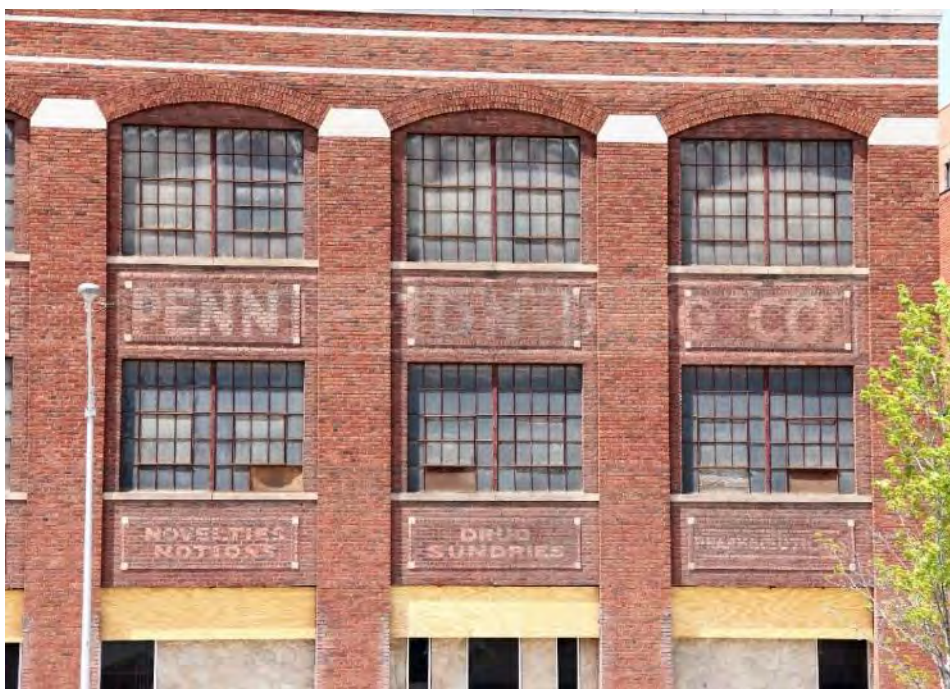
2 of 26: Façade, east wall. Camera facing west.
