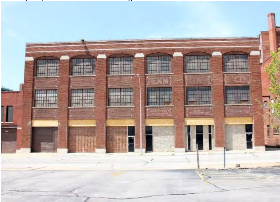
1 of 26: Façade, east wall. Camera facing west.
