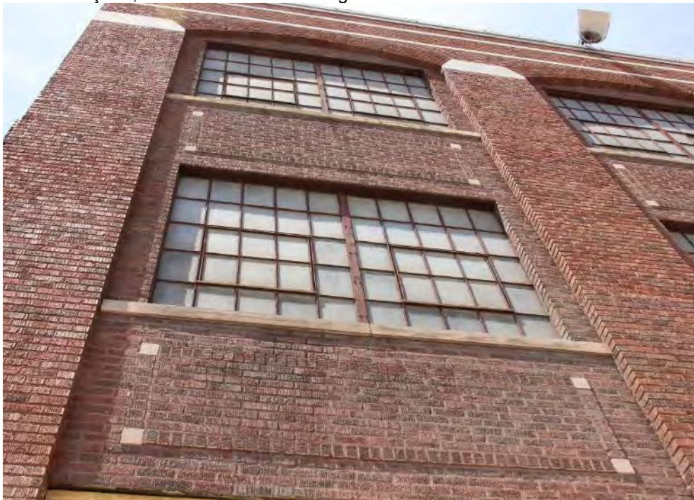
3 of 26: Façade, east wall. Camera facing west.
