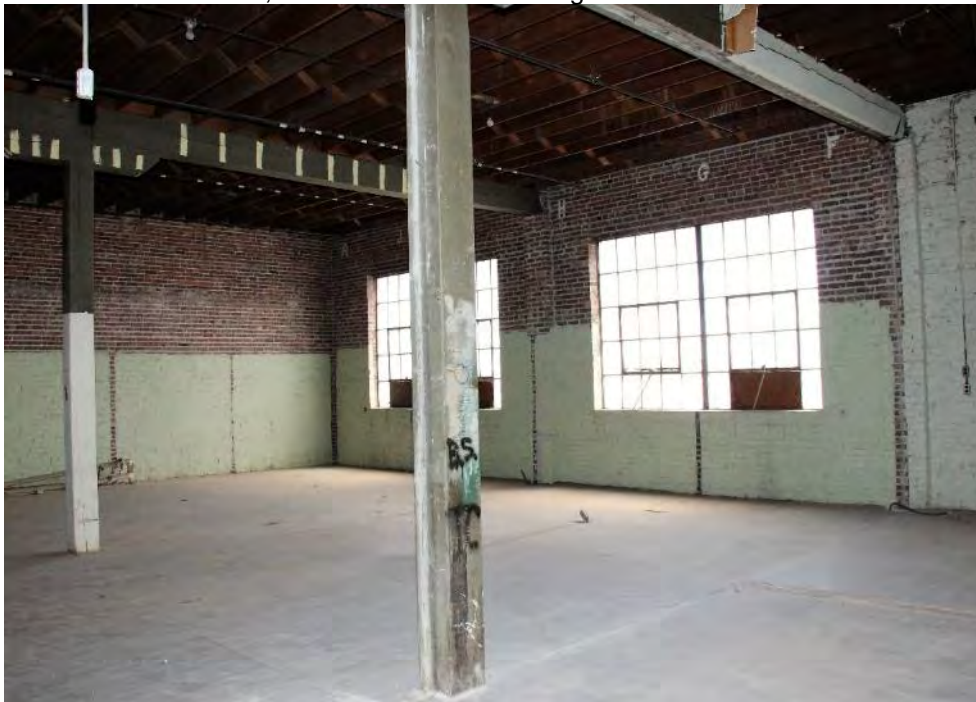
19 of 26: Second floor, north side. Camera facing northeast.
