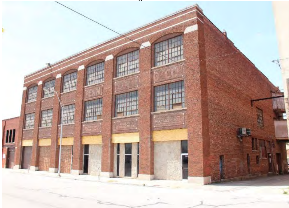
5 of 26: Northeast corner. Camera facing southwest.
