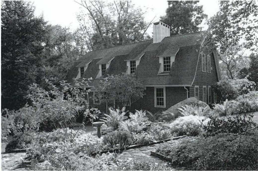
Stepping Stones, main (north) façade, 2008.
