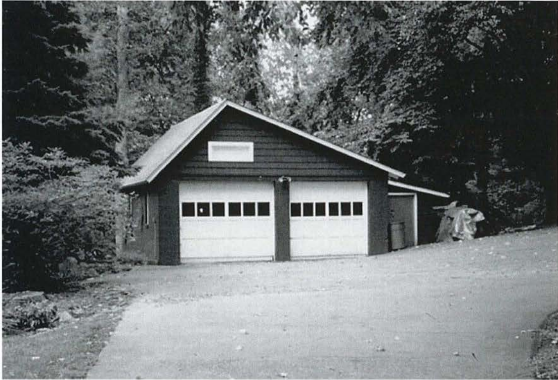
Stepping Stones Garage, constructed 1951, prior to renovation.
